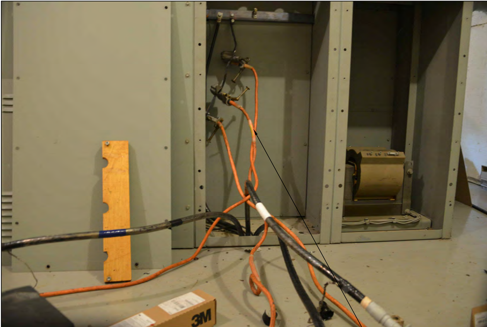
TEMPORARY GROUNDING WORK PRACTICES FOR DISCUSSION
