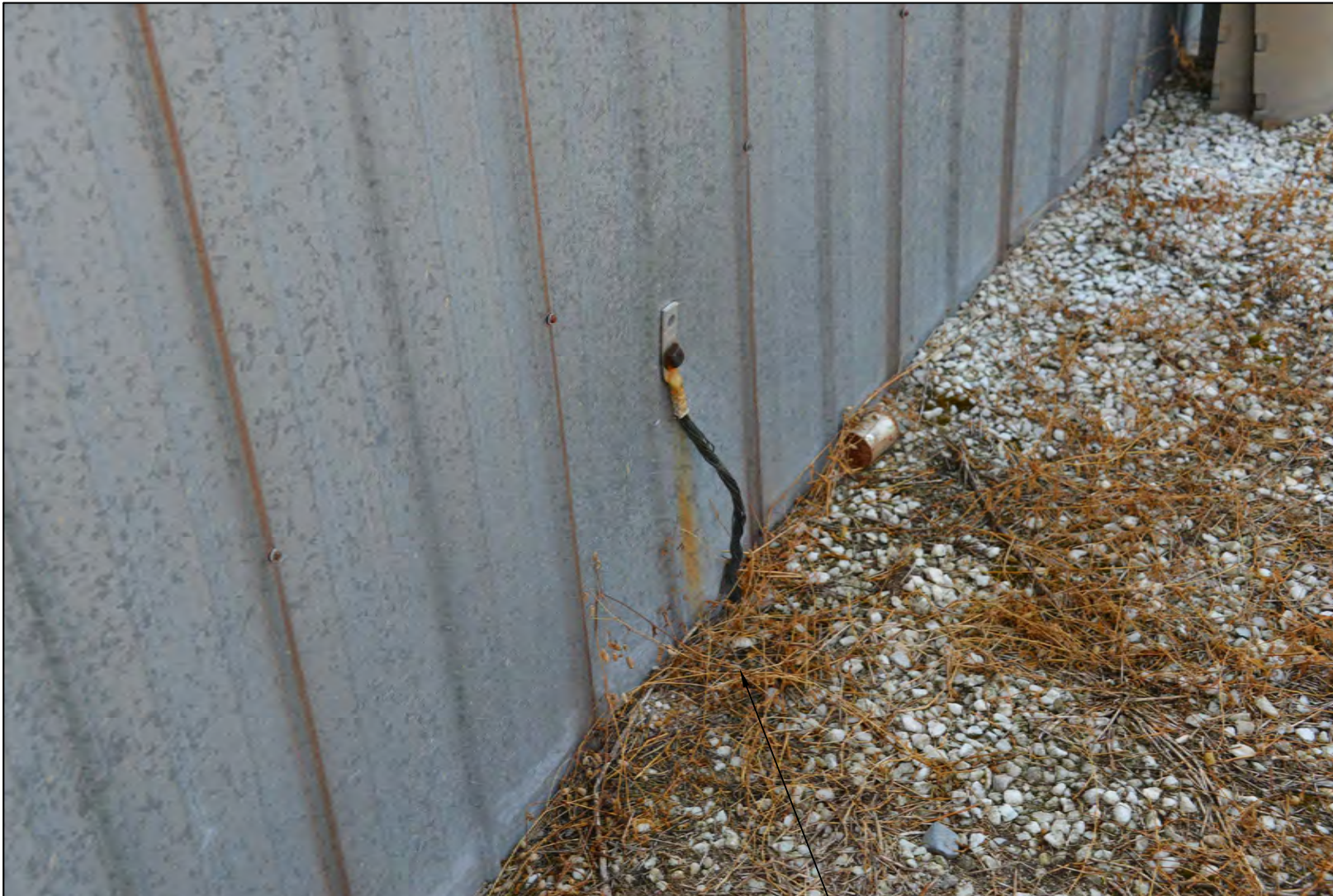
IMPROPER GROUNDING
