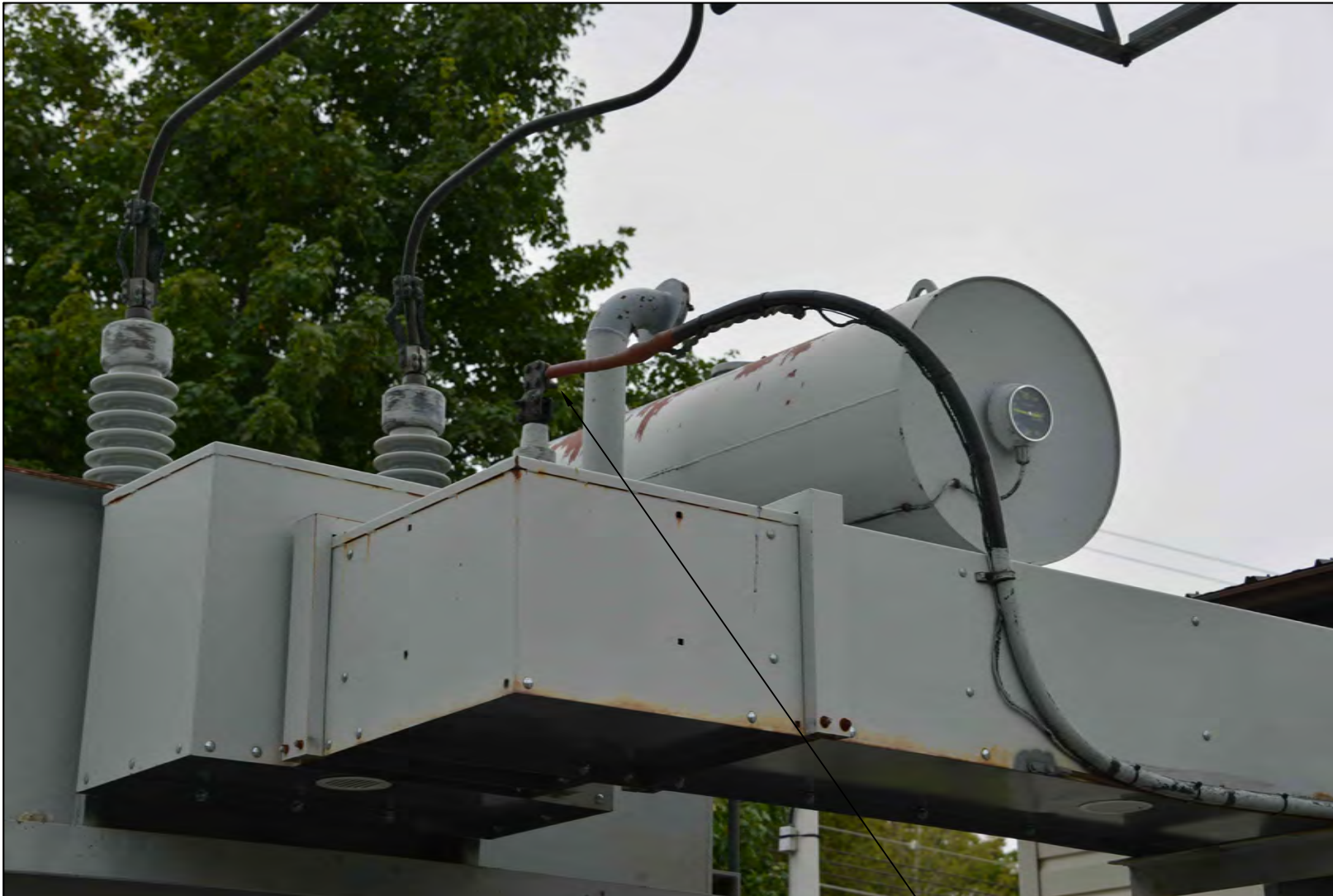
SYSTEM NEUTRAL WITHOUT ANY MECHANICAL PROTECTION
