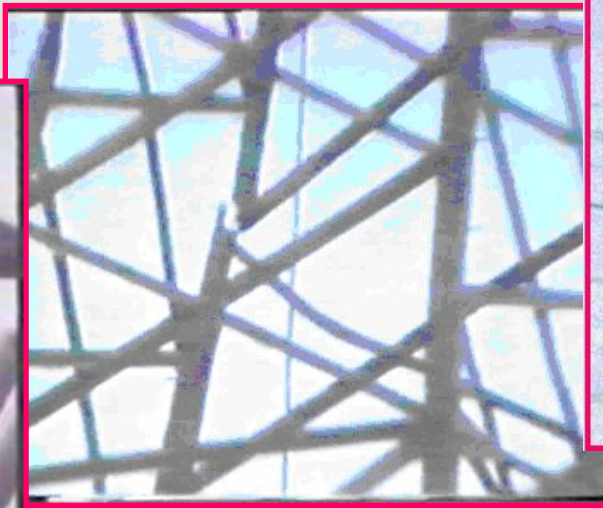
TOWER MAIN LEG BROKEN DURING GALLOPING
