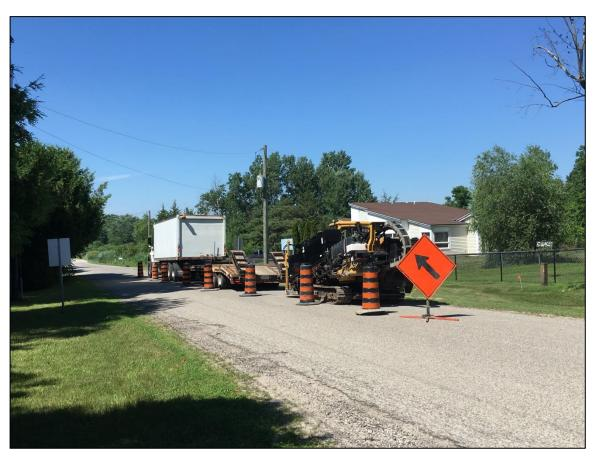
2. At least one lane of traffic was maintained at all times during construction. Flag persons and warning devices were used to notify traffic of construction in accordance with Ministry of Transportation standards.
