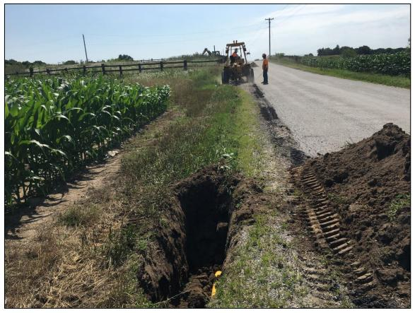
4. Where soil conditions allowed, the pipe was installed via ploughing which further reduced disturbance and potential environmental impacts.
