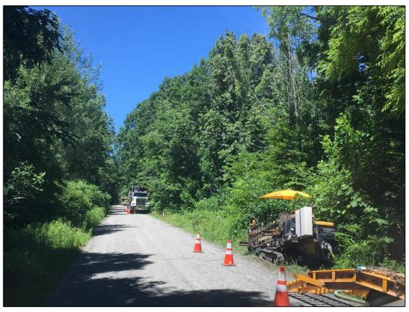
5. The pipe was installed via Horizontal Directional Drilling (HDD) where it was more practical to do so. HDD greatly reduces the amount of tree and vegetation clearing required to install the pipe.
