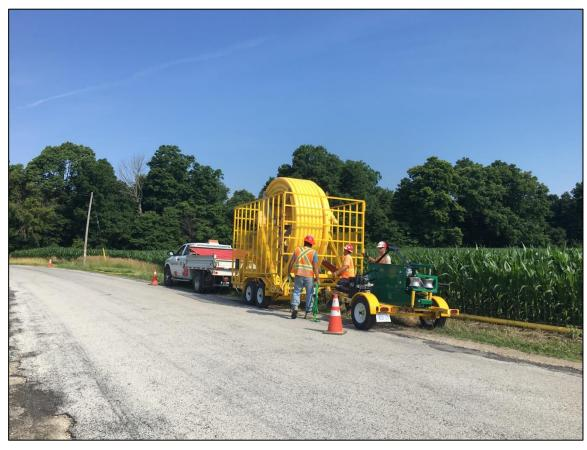
6. The pipeline arrived onsite and was installed off spools.
