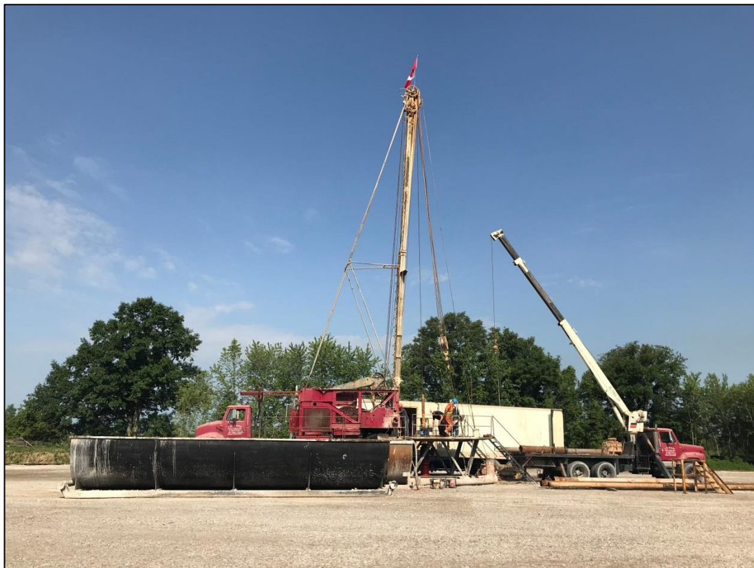
4. Typical well drilling set up on a temporary gravel drilling pad.
