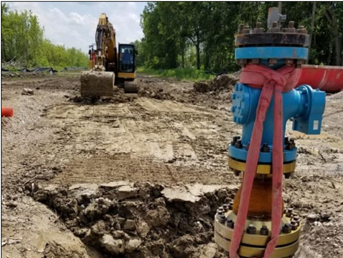
8. Once the new pipeline is installed the topsoil is spread across the work area and seeded.
