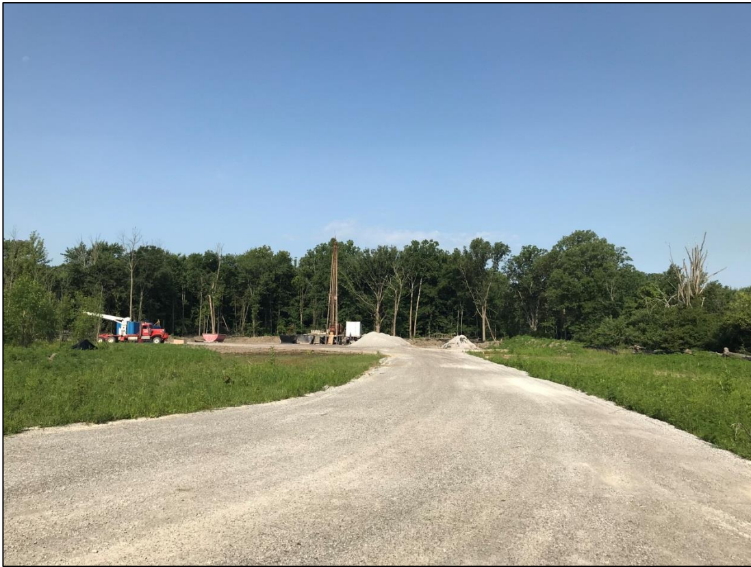
3. Gravel roadways were constructed to provide access to the new wells.
