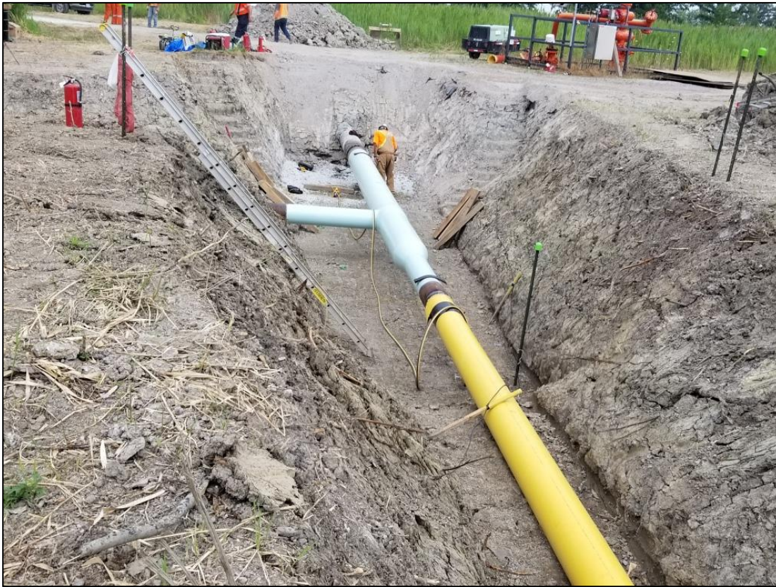
7. The new pipe was connected to the new wells and tied-in to the existing gathering system.
