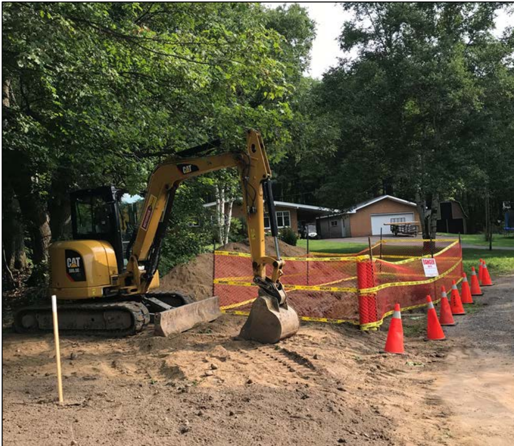
7. All excavations were protected by safety fencing and pylons to ensure public safety.
