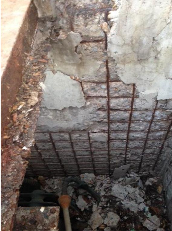
**Figure 3: Crumbling Vault Roof with Exposed Rebar**
