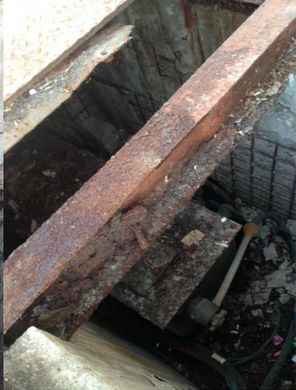
**Figure 4: Corroded I-Beams**
