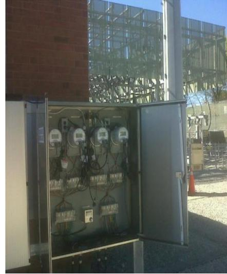
**Figure 15: Wholesale Meter Installation at Transformer Station.**
