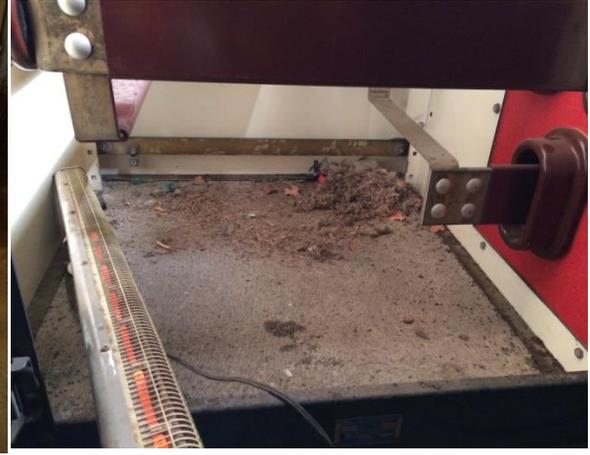
**Figure 16: Pests Inside Outdoor Switchgear**
