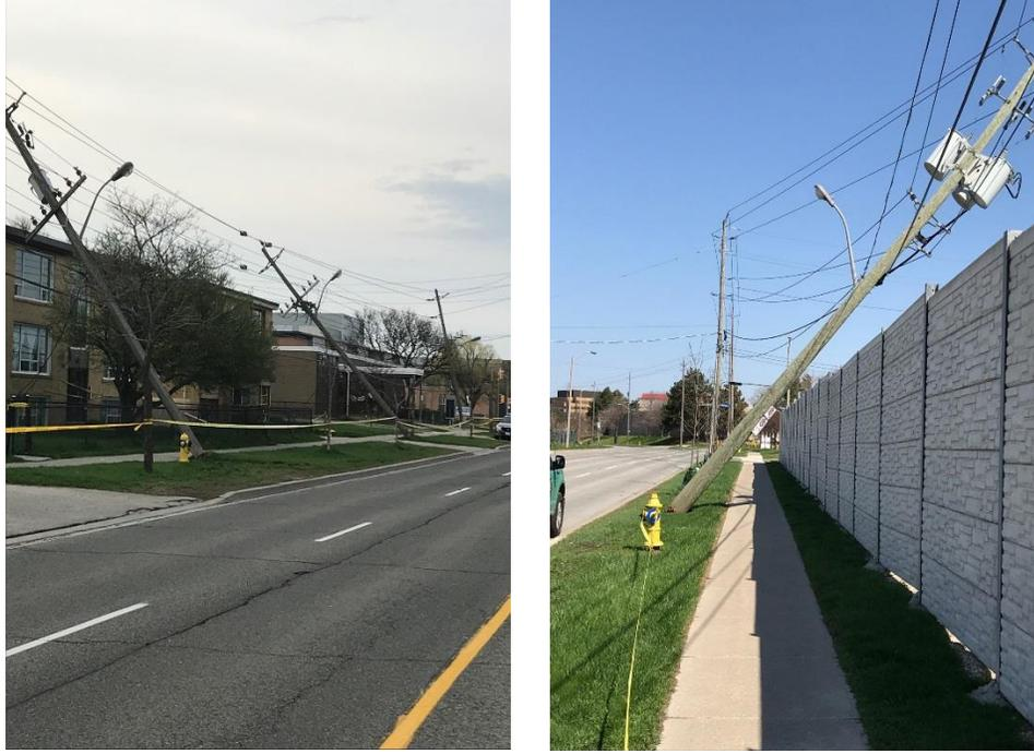
**Figure 6: Examples of Wind Damage Recent 2018 Storm**
