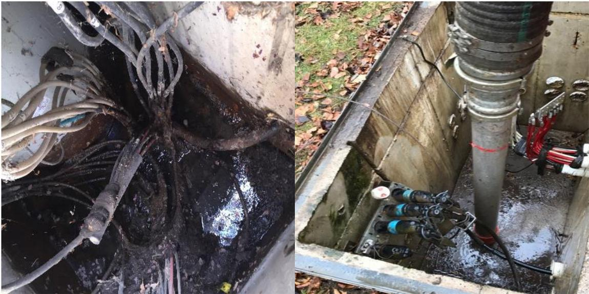
**Figure 8: Oil Leaking from a Transformer
