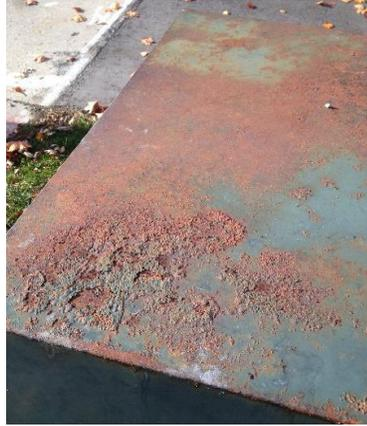
**Figure 15: Padmounted Transformer with Surface Corrosion**
