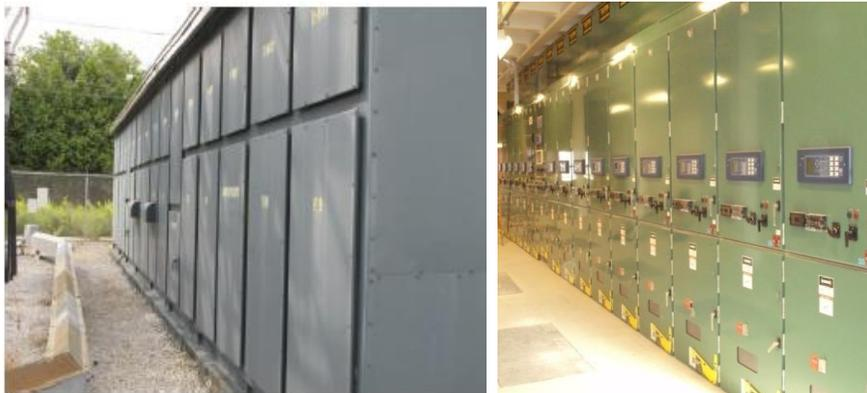
11 **Figure 13: (Left) Outdoor Enclosure Housing Metal clad Switchgear. (Right) Indoor**
