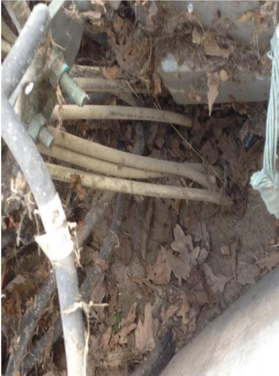
**Figure 6: Vault Full of Dirt and Debris**
