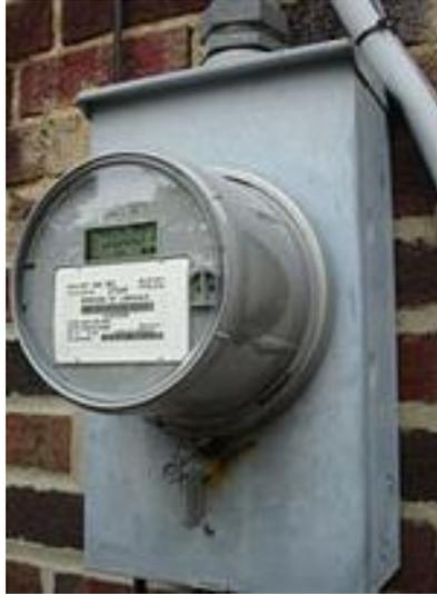
**Figure 14: Smart Meter Installation at Customer Location.**
