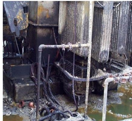
**Figure 25: Leaking Fluids from Failed Transformer**
