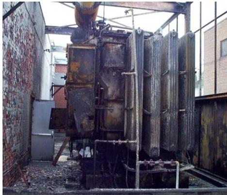
**Figure 24: Damages to the MS Wall**
