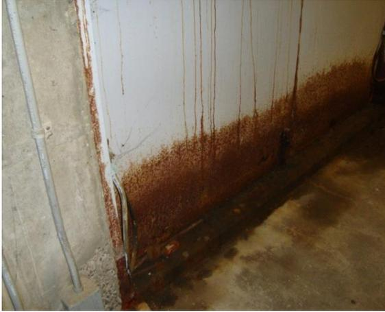
**Figure 15: Rusted Switchgear Enclosure**
