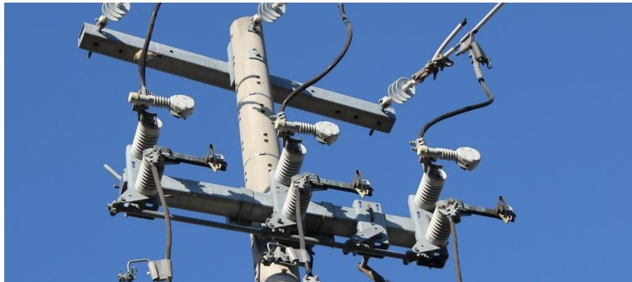
**Figure 6: Manual Gang-Operated Switch**
