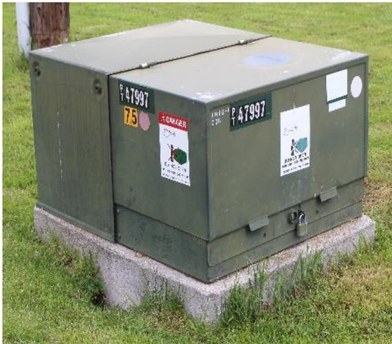
**Figure 11: Padmounted Transformer**
