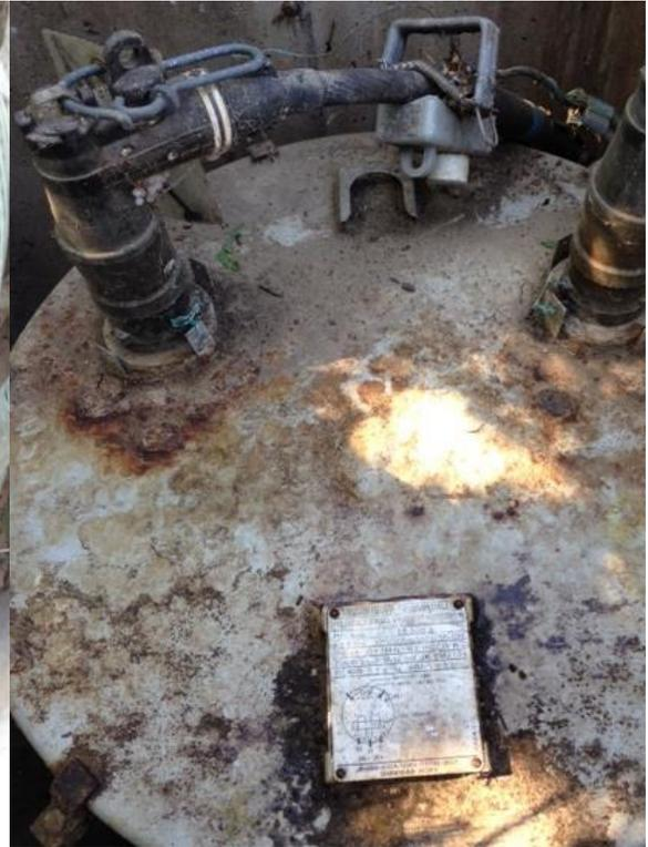
**Figure 7: Corrosion on Top of a Transformer**
