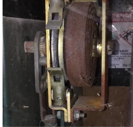
**Figure 16: Padmounted Switch with Rusted Coil Spring**
