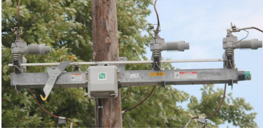
**Figure 5: SCADA-Mate Switch**
