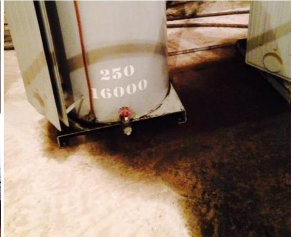
**Figure 3: Transformer Leaking Oil**
