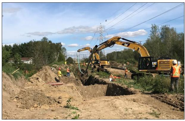
6. When crossing a watercourse, a shorter section of pipe is welded together to be able to complete the crossing as quickly as practical to minimize potential impacts.
