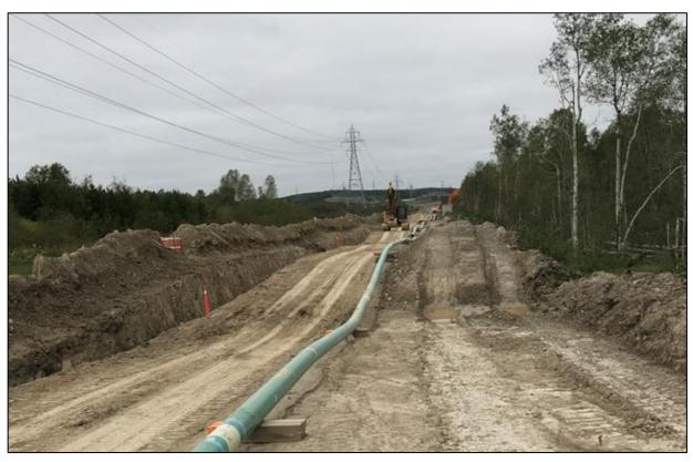
4. Once the trench for the new NPS 12 was dug, the pipeline was strung out parallel to the trench and welded and coated in preparation to be lowered-in.
