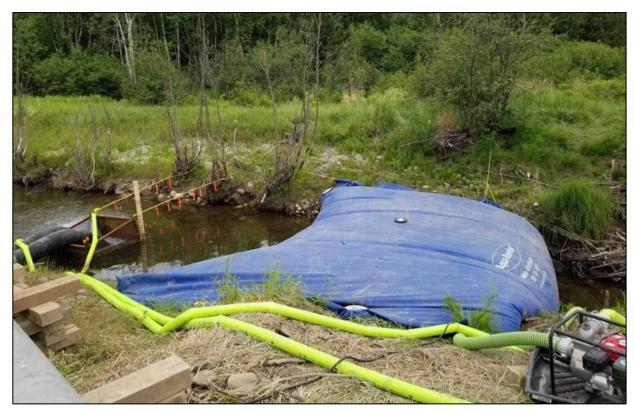
5. A number of watercourses were crossed during pipeline construction using Union's Fisheries and Oceans Canada – approved Dam & Pump method. Permits from the local Conservation Authority and Ministry of Natural Resources and Forestry were also obtained and adhered to.
