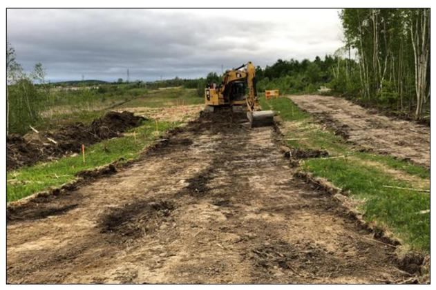
1. Topsoil is stripped from the right-of-way and separated from subsoil during pipeline construction to ensure vegetative growth after restoration.
