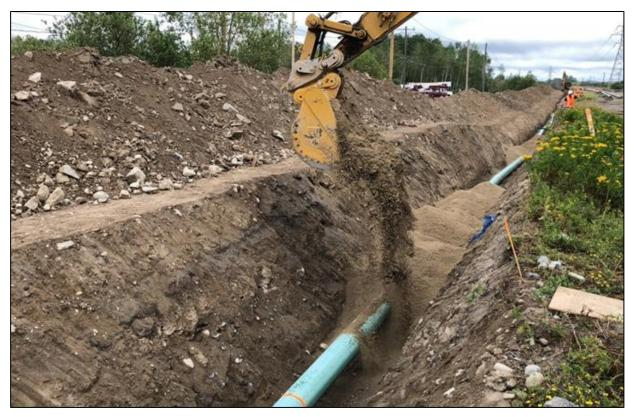
7. In areas with rocky soils, the pipe is covered with sand prior to backfilling with native material to prevent damage to the new pipe.
