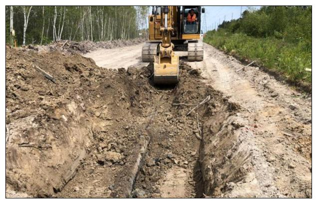
3. After the topsoil was stripped and the right-of-way was graded, the existing NPS 10 pipeline was excavated and removed.
