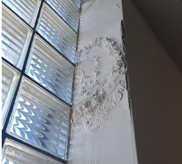
Figure A17 - 2: Water Damage Nebo Road Roof
