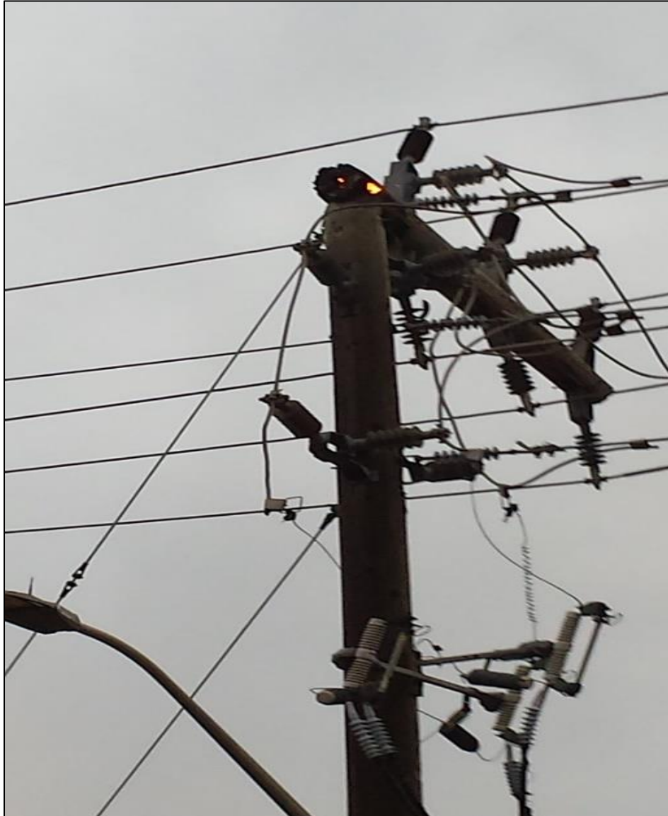
Figure 5.3.3 - 22: Active Pole Fire Event Alectra Utilities
