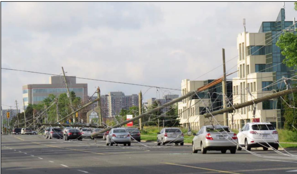
Figure 5.3.3 - 17: Downed Overhead Line on Warden Avenue in Markham on June 17, 2014
