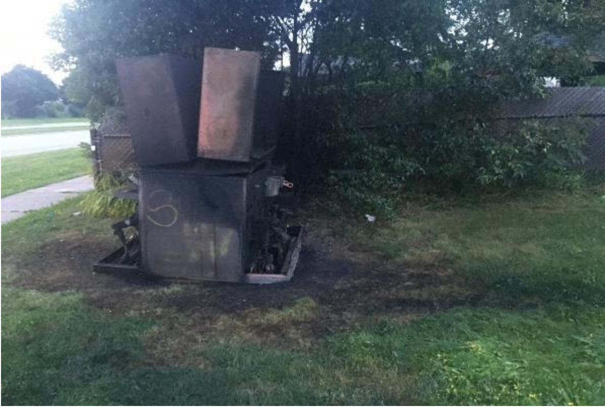
Figure A10 - 15: Failed Oil-Filled Switchgear, August 2018
