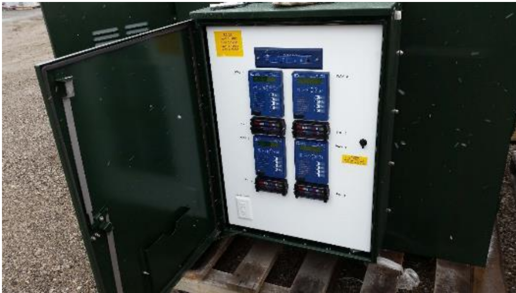
Figure A10 - 25: Automation Cabinet on Switchgear
