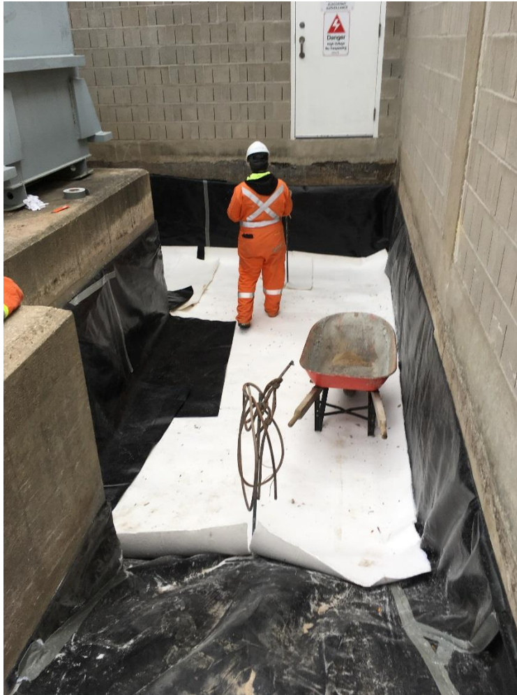
Figure A15 - 1: Sorbweb Installation
