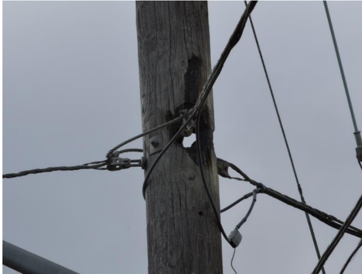
3 Figure A05 - 12: Wood Pole Fire Resulting from Tracking Insulators
