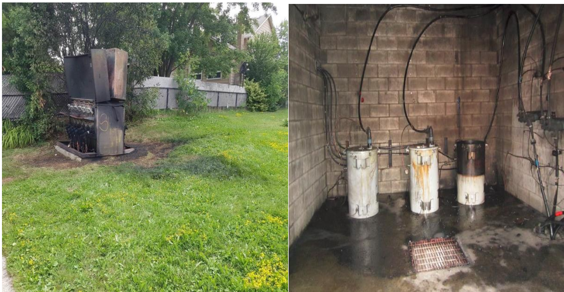
Figure A06 - 1: Catastrophic Failure of Switchgear and Vault Transformer
