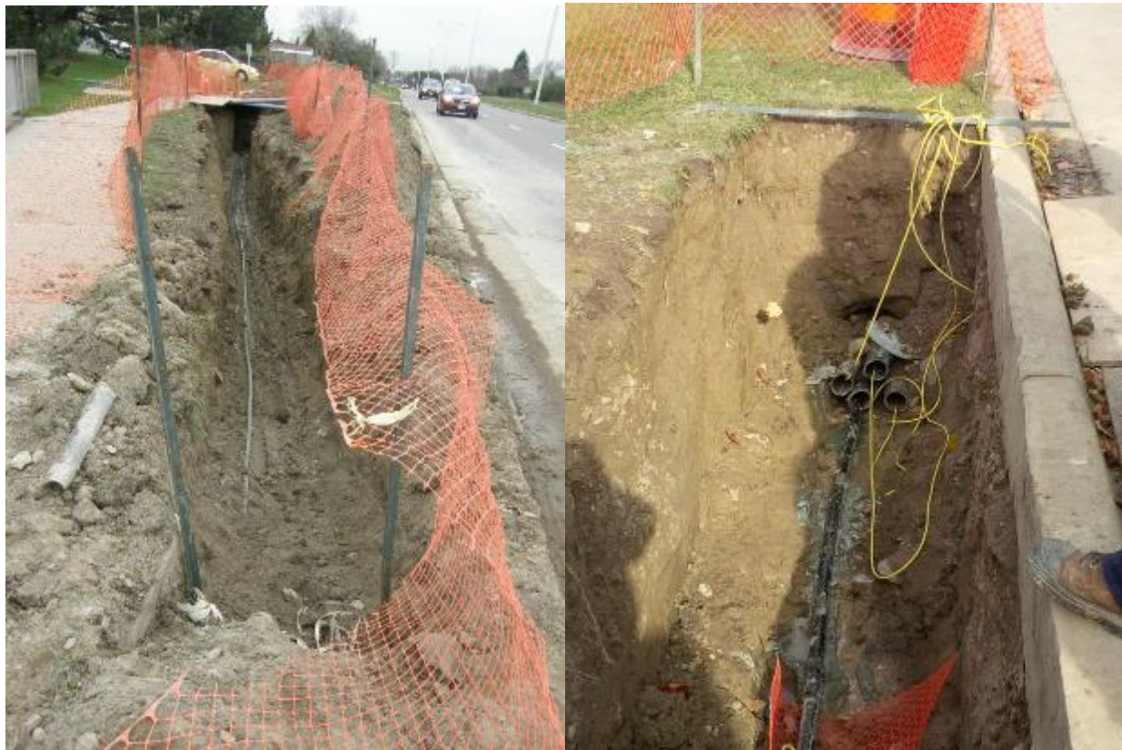
Figure A10 - 4: Underground Cable Replacement
