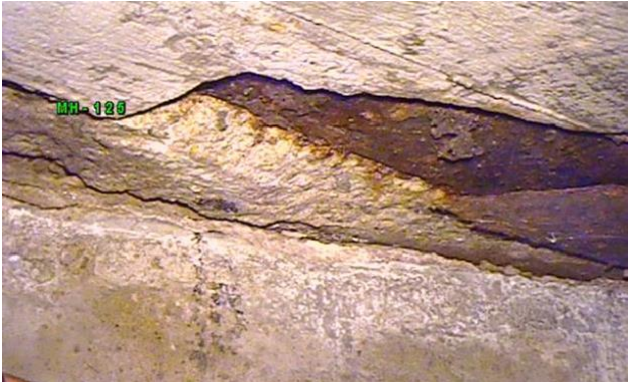
Figure A10 - 29: Lid Degradation: steel supporting rusting
