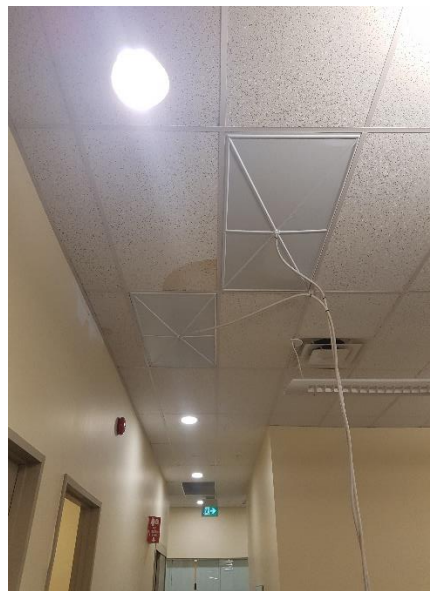
Figure A17 - 2: Water Damage Nebo Road Roof
