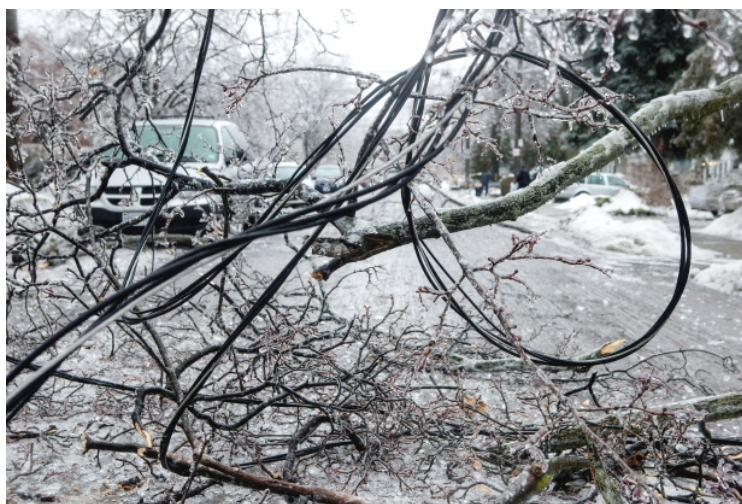
FIGURE 3: FALLING BRANCH ON STREET ENTANGLED WITH CONDUCTOR 3
