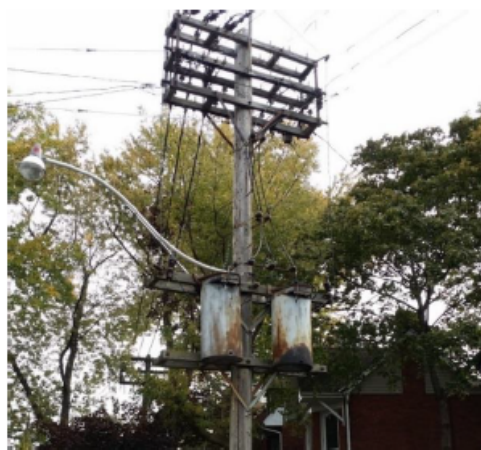
Figure 4: Box Construction in a Backyard with Leaking Equipment
