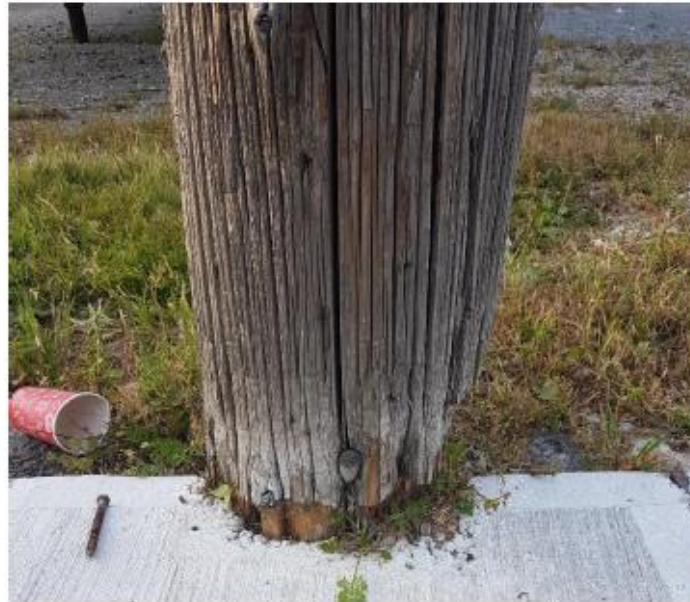
Figure 12: Deterioration at the base of a pole
