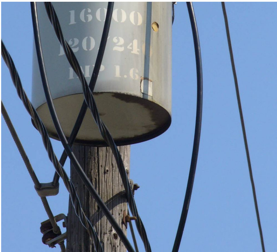
Figure 17 Transformer with Minor Rust
