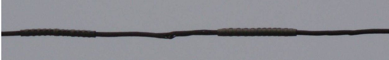
Figure 16 Conductor in Poor Condition
