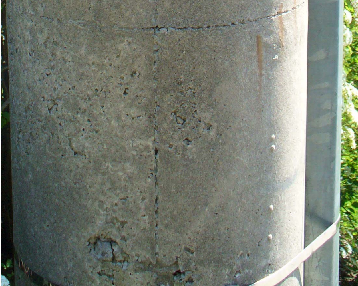
Figure 15 Concrete Pole with Exposed Aggregate
