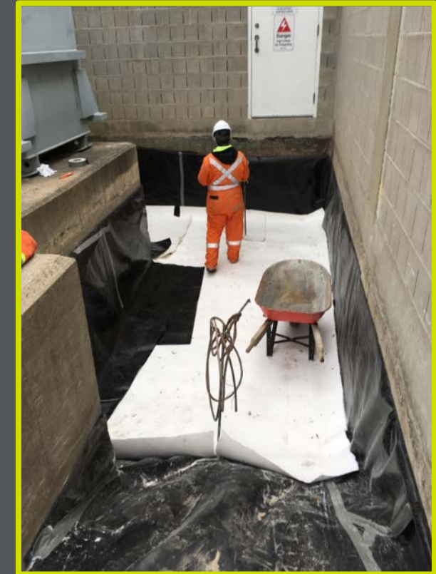
Installation of Oil Containment Solution
