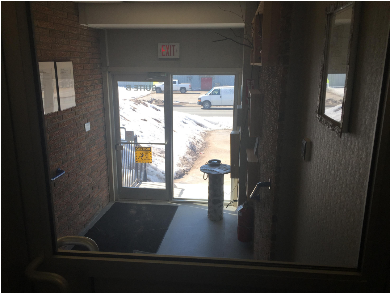
Suite 'B' First Floor Photo 21 – Photo of the entrance vestibule from Sackville Road.
