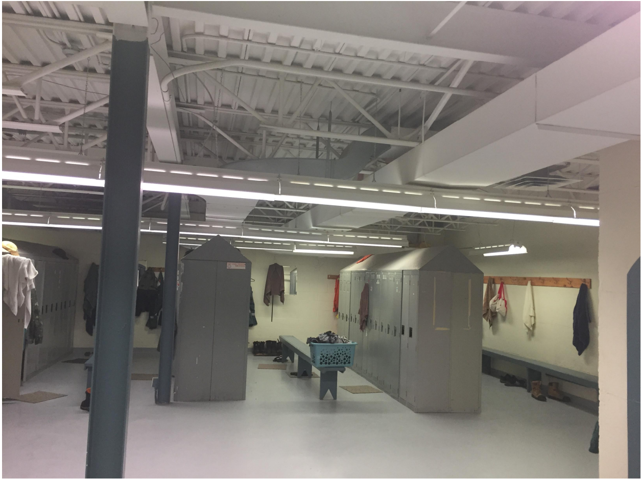
Suite 'B' Basement Photo 5 – Men's washroom / change room / shower.
