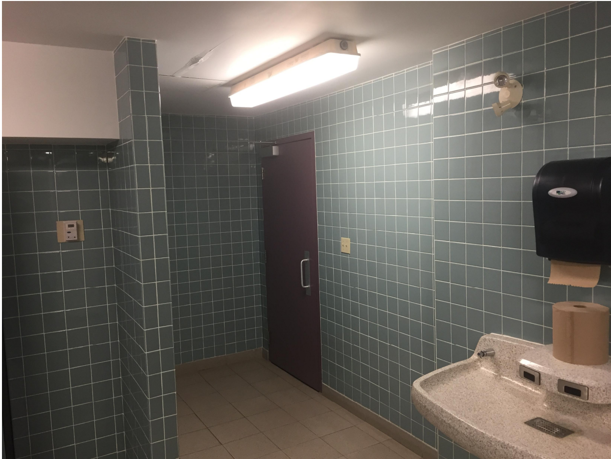
Suite 'B' Basement Photo 2 – Entrance to Woman's washroom / change room / shower.
