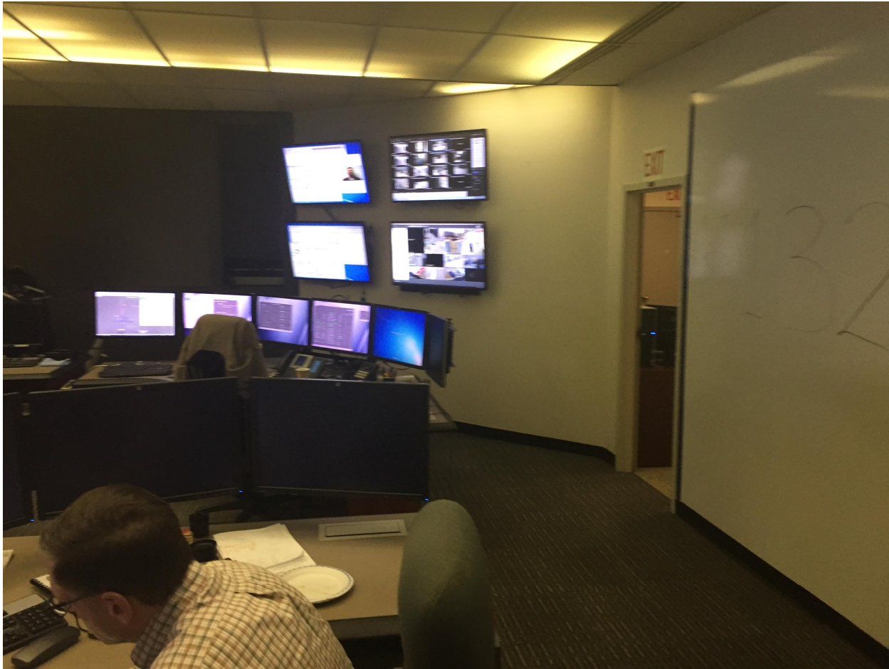
Suite 'B' First Floor Photo 22 – Photo of the control room. The equipment and services undertaken within this room are beyond the scope of this document.
