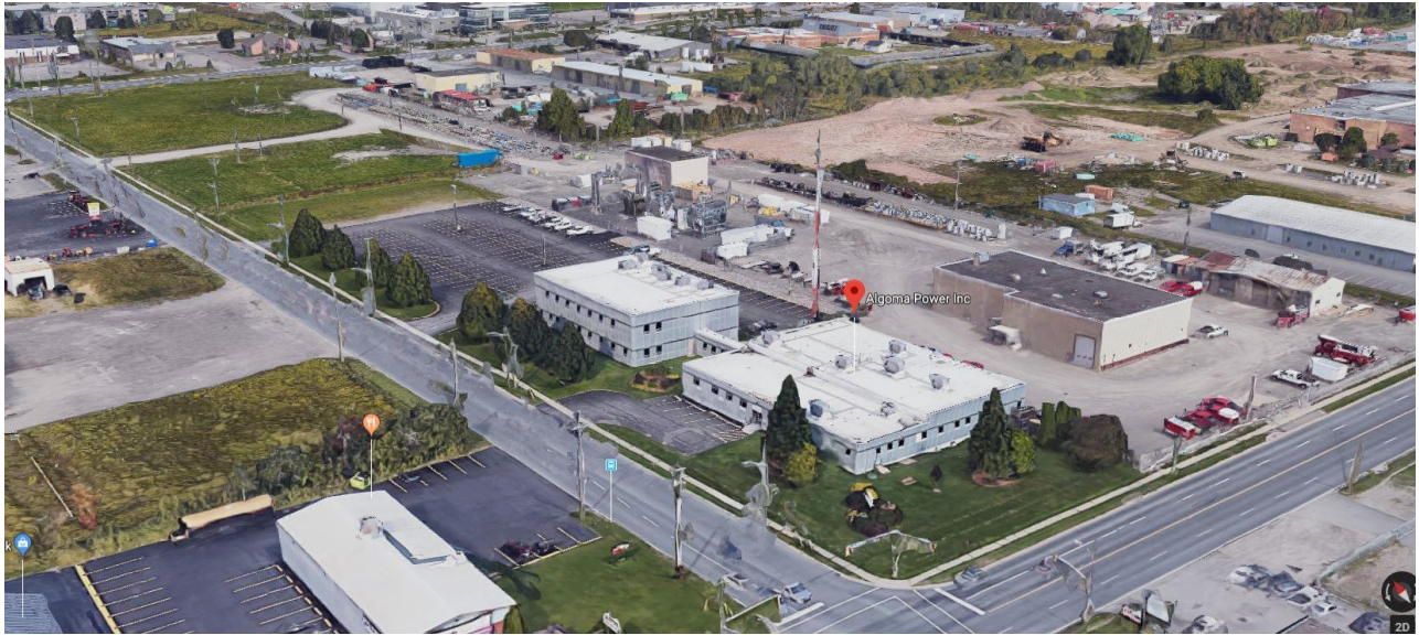
General Facility / Complex - Photo 1 – Aerial 2 Sackville Road – Looking North East
