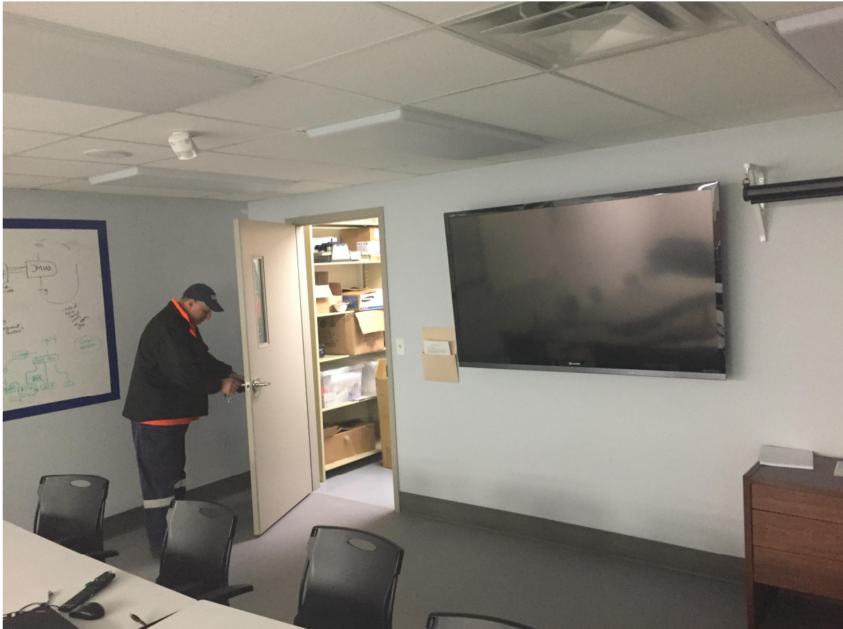
Suite 'B' Basement Photo 14 – Photo of typical basement conference room. Note hollow metal doors and frames mounted into steel stud and gypsum board partition walls. Also S.A.T. can be noted as the ceiling finish. This room contains Vinyl sheet flooring (Montreal room).
