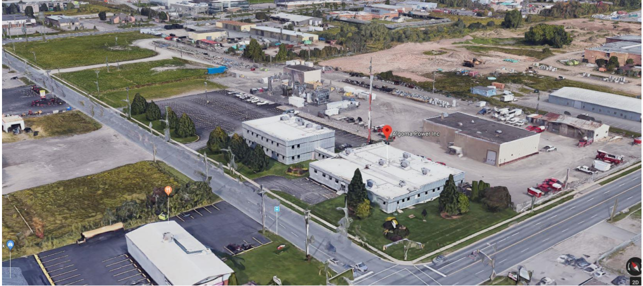
General Site Photo 1 – Aerial 2 Sackville Road – Looking North East
