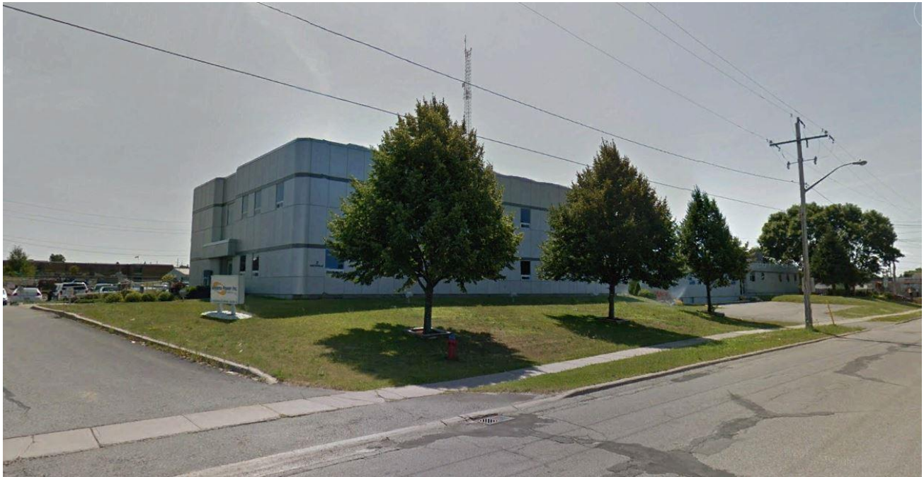
Exterior Photo – Looking South East, viewed from Sackville Suite 'B'
