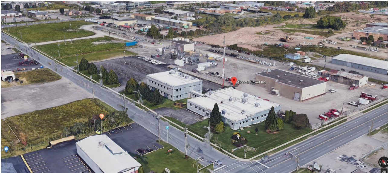
General Site Photo – Aerial 2 Sackville Road – Looking North East
