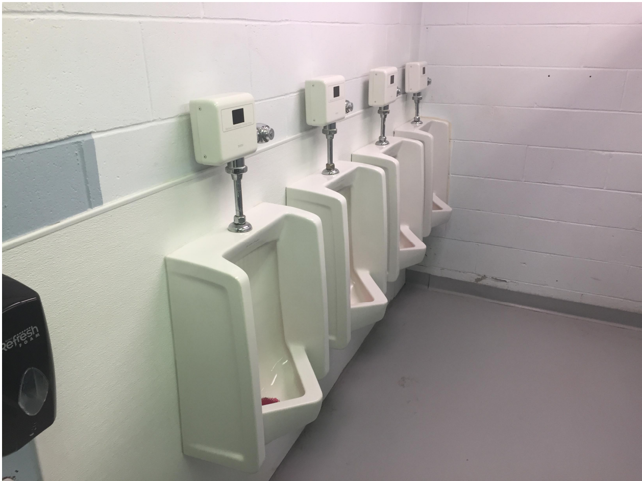
Suite 'B' Basement Photo 6 – Men's washroom / change room / shower.
