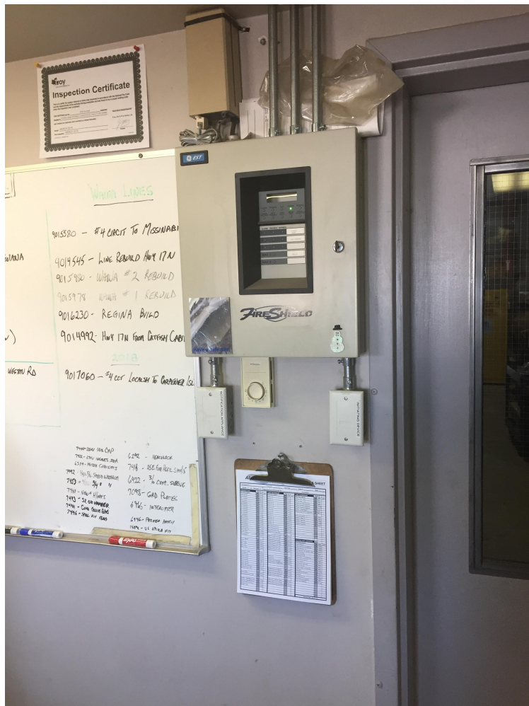
Stores Photo 3 – Entrance door from the office addition into the open storage space. Note the fire alarm and thermostat. The thermostat controls a 4' baseboard heater.
