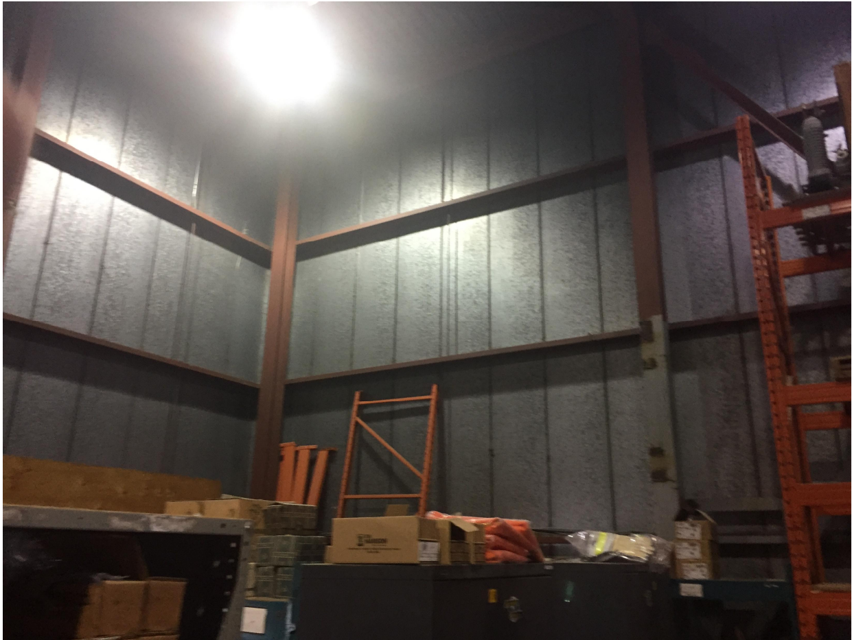
Stores Photo 4 – General structural framing and interior view of the exterior vertical metal siding, c/w channel girts.
