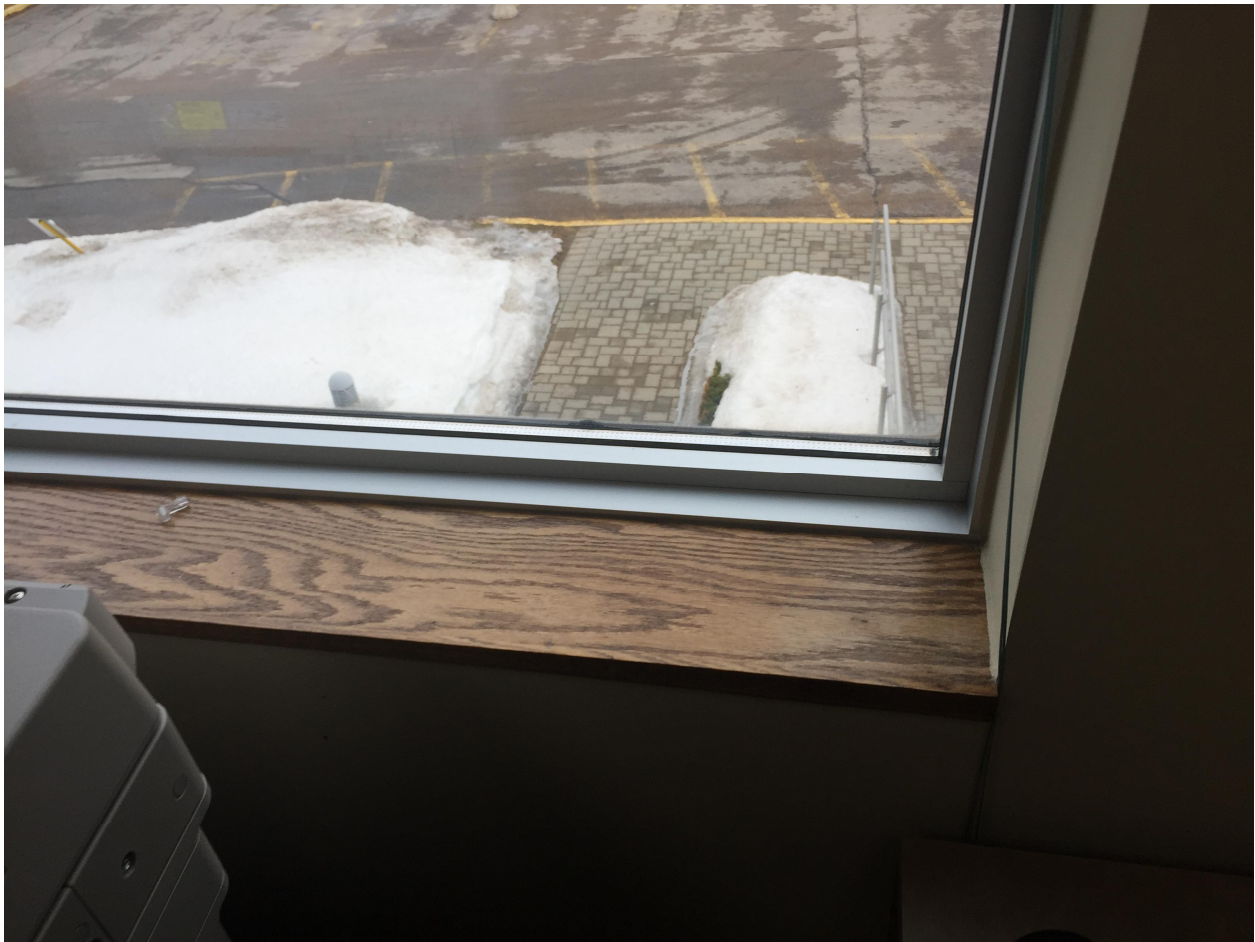
Suite 'A' Photo 15 – 2 nd Floor – Looking North. The window sills, jambs and headers show little to no damage due to the earlier issues describe in Photo 8. This may be due to the amount of water on the wall or the general placement of the aluminum panels. Regardless of the lack of visible damage the protocol described in photo 8 should be carried out throughout the main and 2 nd floor. (API)
