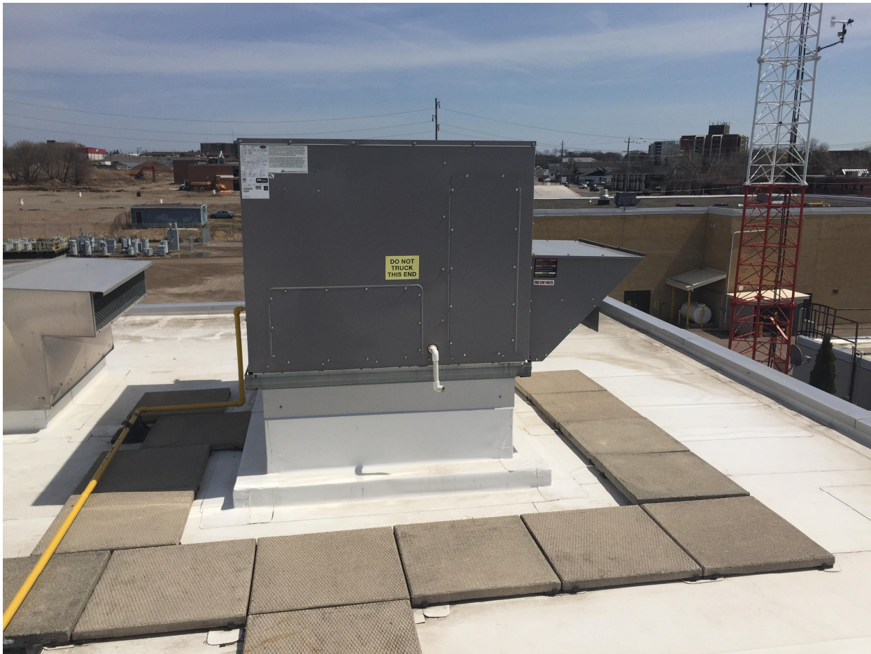
Suite 'A' Photo 29 – Typical Roof Top Unit (RTU) Suite 'A'.
