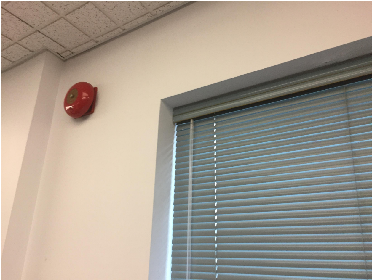
Suite 'A' Photo 13 – View of a fire alarm bell. It was noted that there were several bells located throughout all floors. As well fire extinguishers and pull stations were also noted at appropriate locations. Discussions with maintenance staff confirmed that the system is regularly tested and certified. (API)
