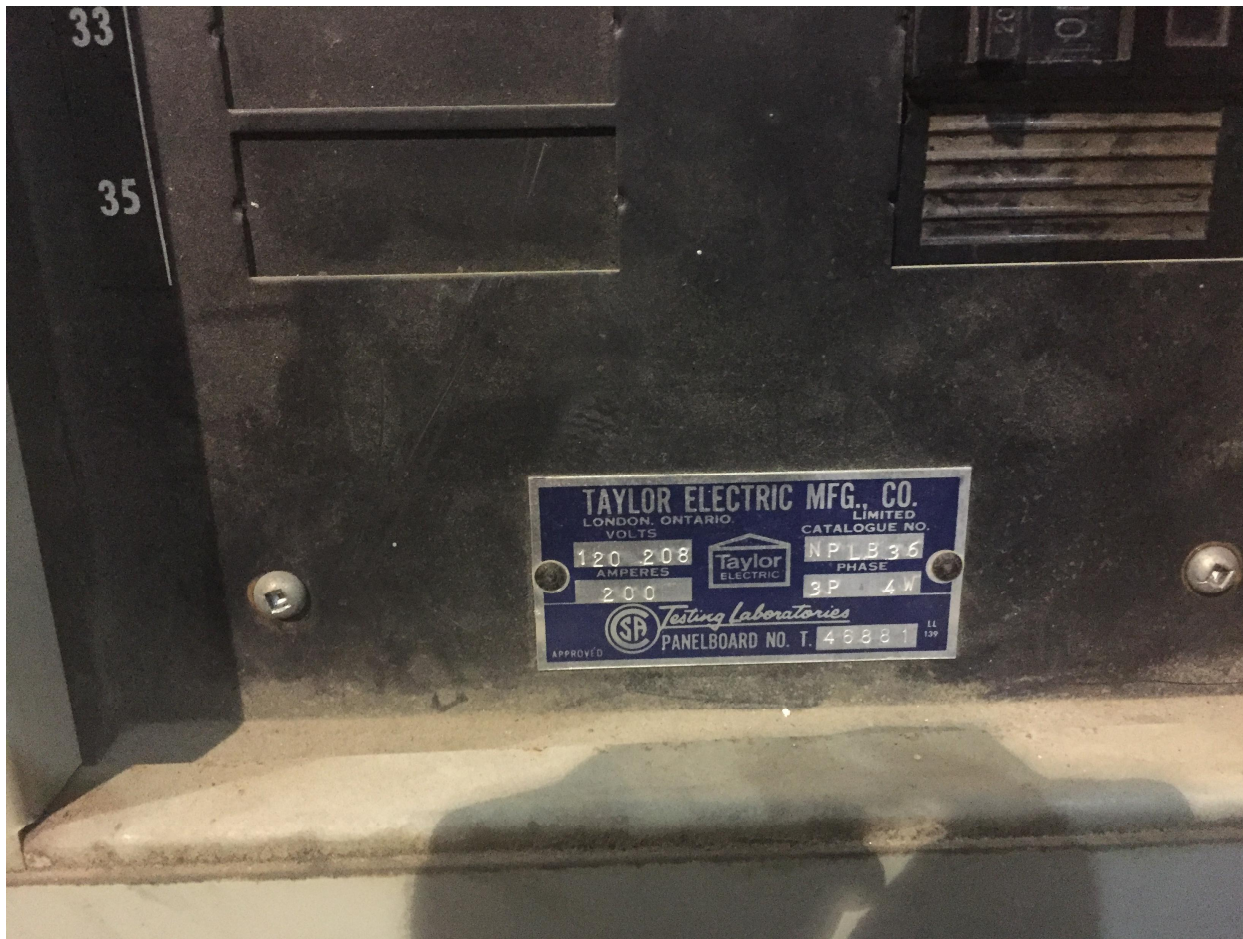
Stores Photo 9 – Photo of one of the two electrical panels. There are 2 – 200amp, 120/208v panels.
