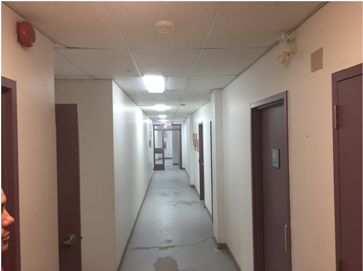
Suite 'A' Photo 21 – Basement. Typical corridor. The main floor finish is paint on concrete. Some paint is spalling due to a minor flood. After discussions with maintenance staff the floor is scheduled to receive new paint in the future.
