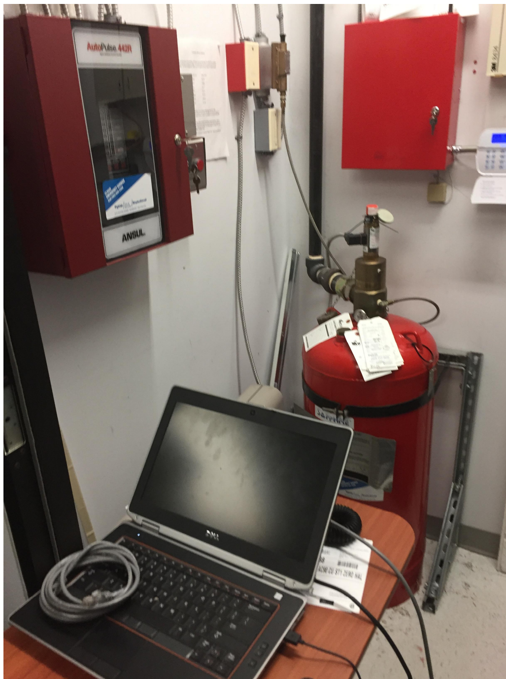
Suite 'A' Photo 19 – 2 nd Floor – Computer server and IT office. The afore mentioned room is served by a Dry Chemical Suppression and alarm system. This system is regularly reviewed and certified by an approved agency.
