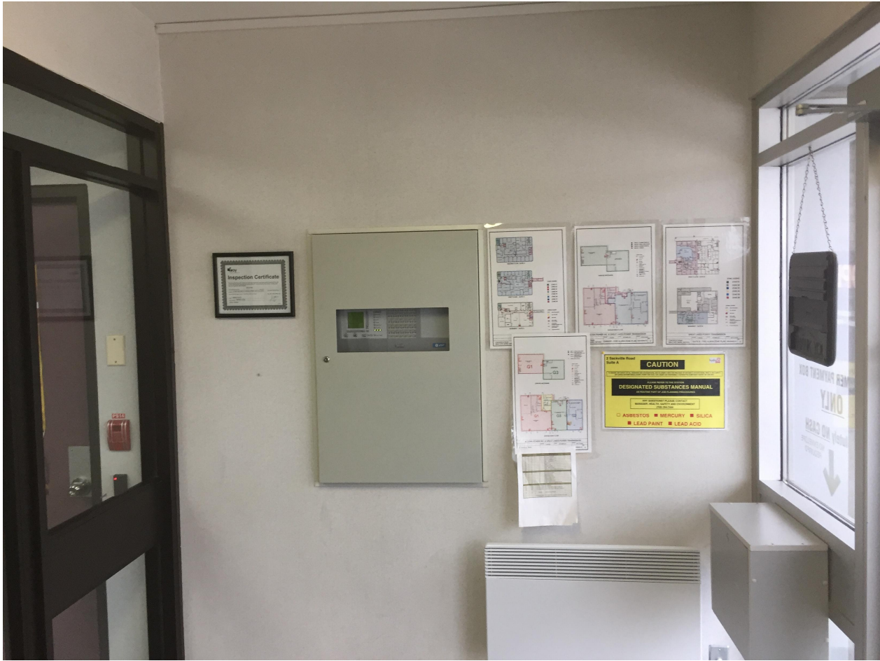
Suite 'A' Photo 6 – Main Floor Vestibule / Fire Alarm Station – Annunciator Panel. (API)
