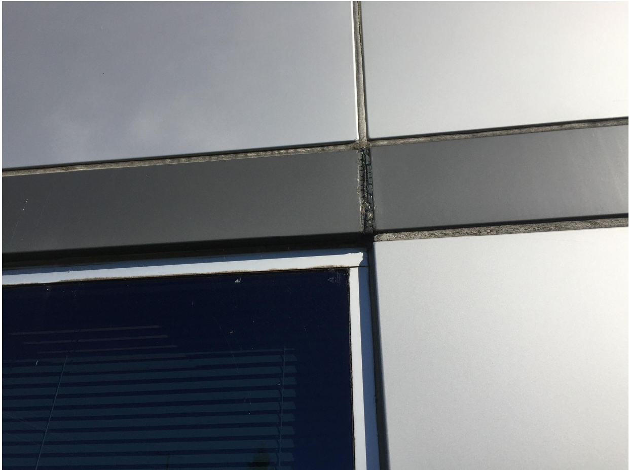
Suite 'A' Photo 8.1 – Exterior view of the exterior aluminum panel system and caulking failure. A coloration seemed to exist between the accent band (brown color panel) and the location of leaks. It may be apotheosized that the color of the caulking or its chemical makeup was not as resilient as the lighter shade of caulking.
