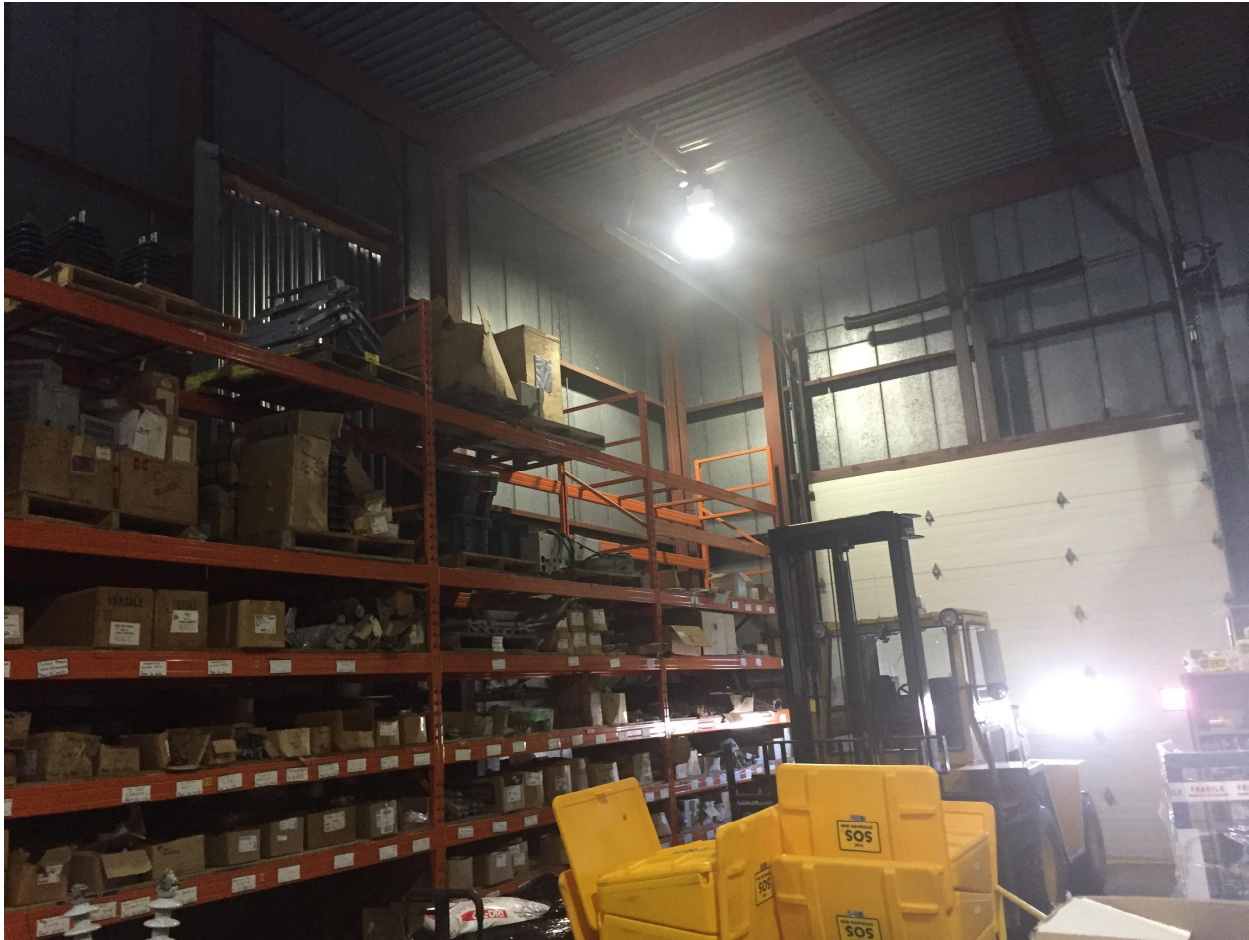
Stores Photo 5 – General structural framing and interior view of the exterior vertical metal siding, c/w channel girts as well as interior pre-engineered shelving units. OH 12'w x 14'h door complete with electric and manual operator.
