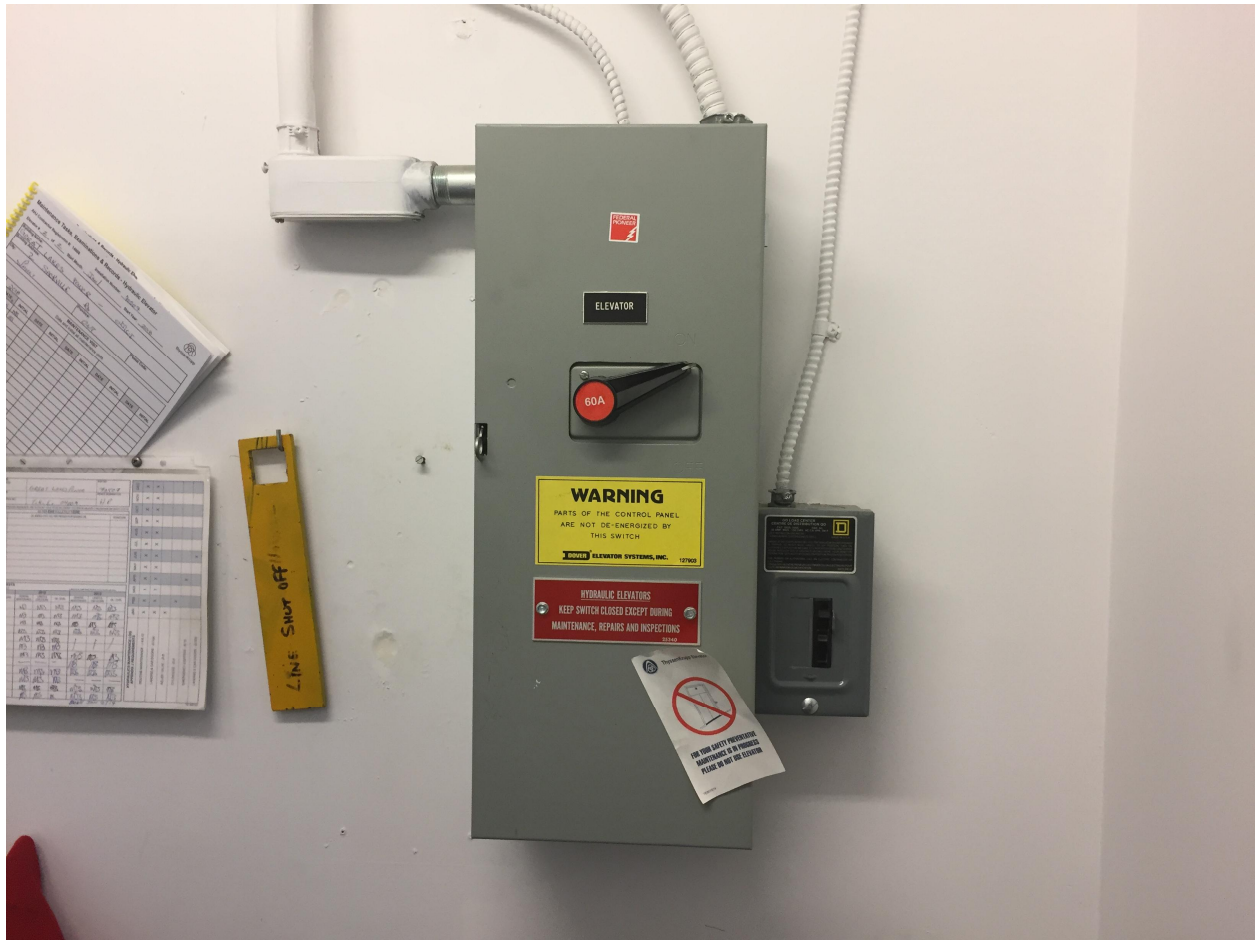
Suite 'A' Photo 25 – Basement. Elevator main disconnect switch.
