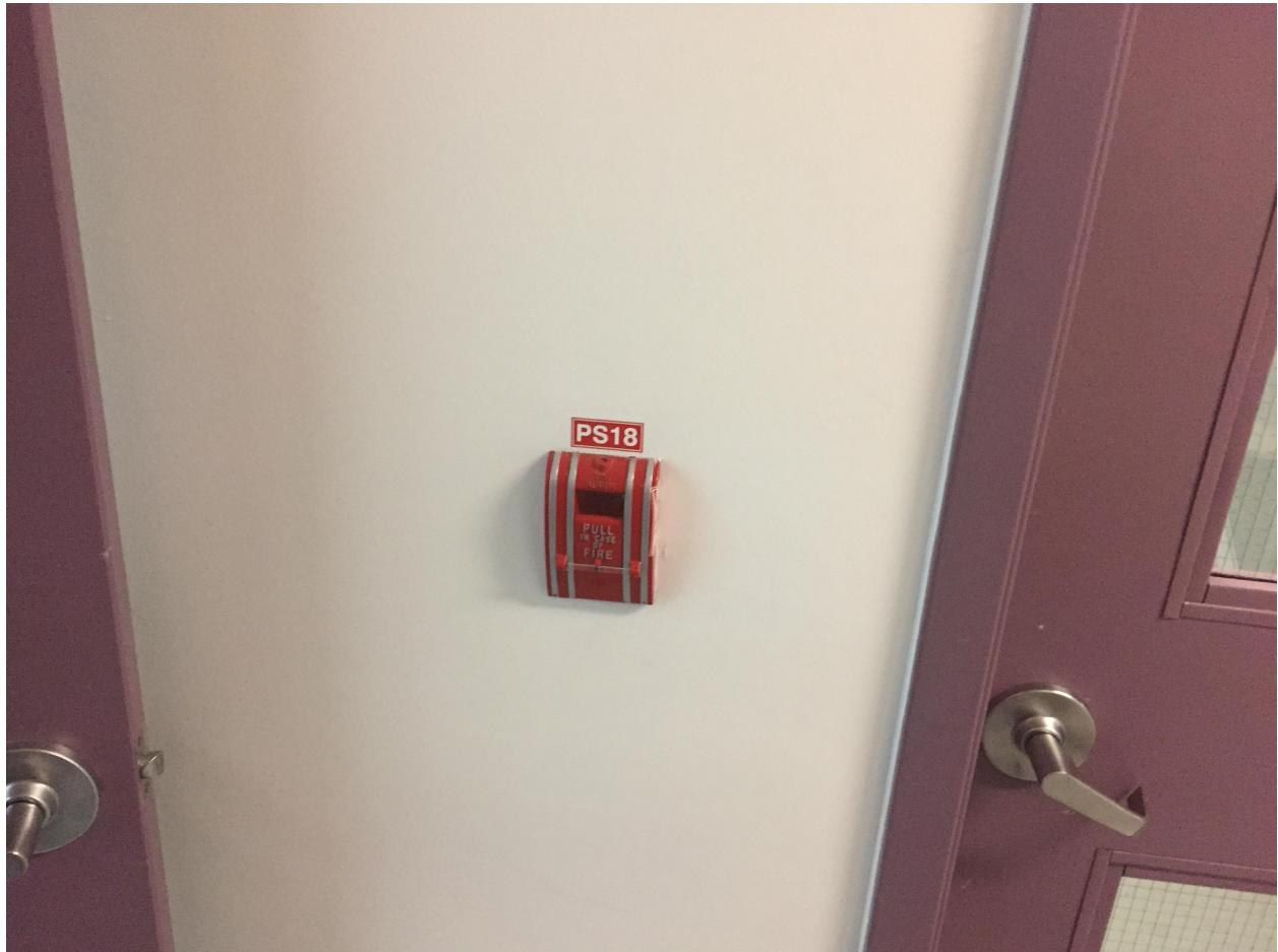
Suite 'A' Photo 20 – Basement. Typical fire alarm pull device. These items are located throughout the facility and appear to be located at the appropriate locations. All locations can be found on archived drawings from the mechanical / electrical engineer on the original building drawings. (API)
