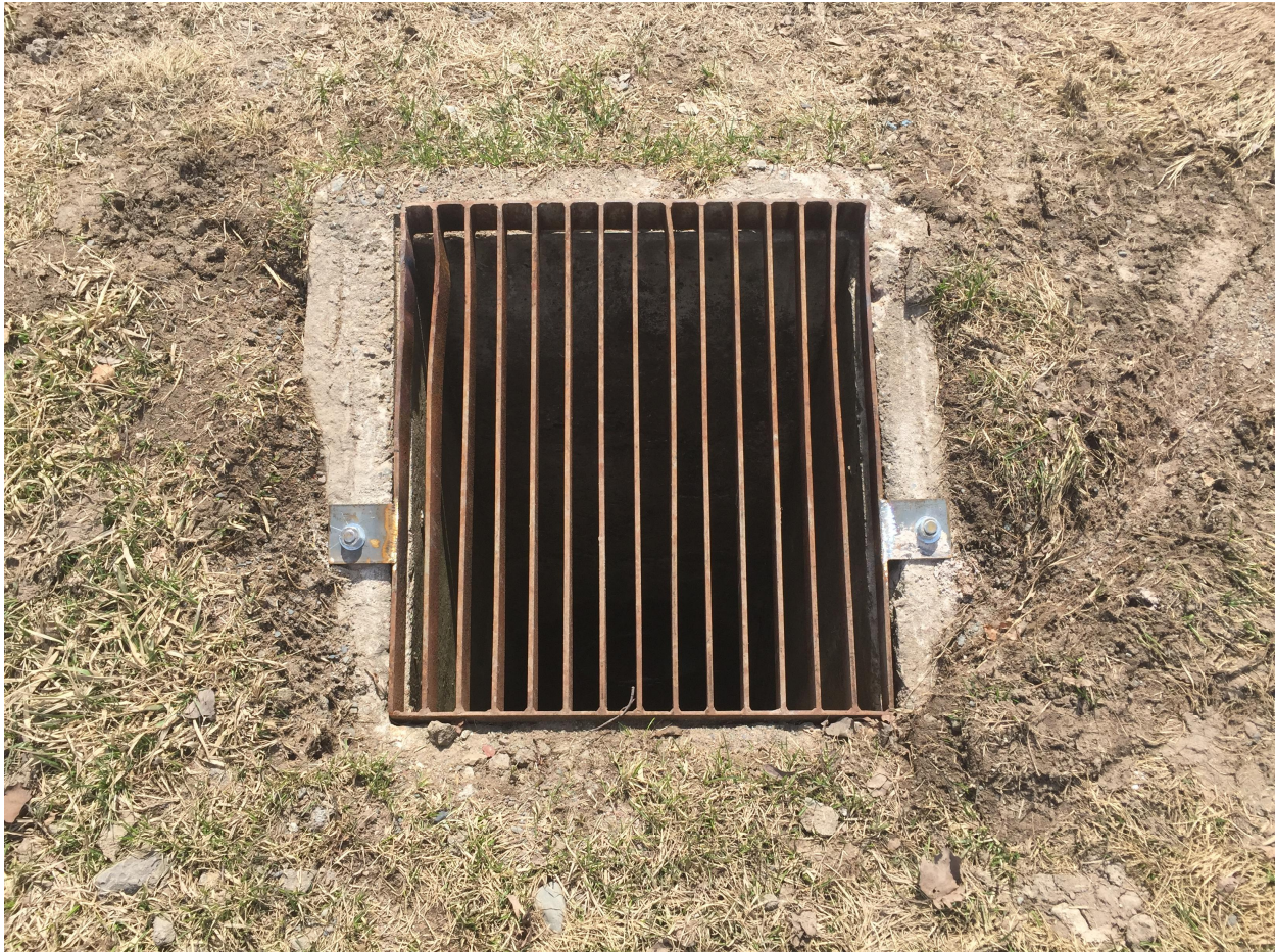
General Site, Photo 4 – Ditch Inlet Catch Basin – This structure is located at north side of the second entrance to the main parking area. The main parking area catch basins drain to this basin. It then is fully entered into the City of SSM storm water system.
