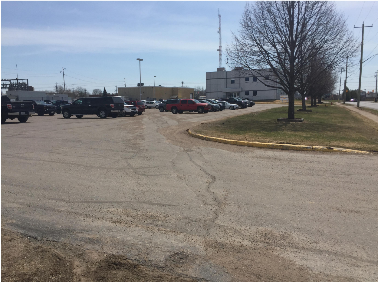
General Site, Photo 6 – Second Entrance of Main parking area – Looking South. There is obvious settlement of the soils of the parking area around the main storm drain.
