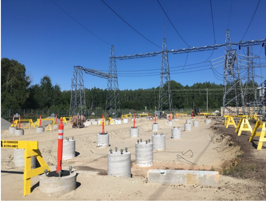
Wawa TS – Civil and foundation work underway
