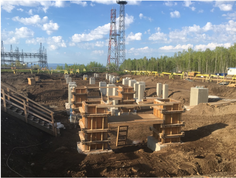
Lakehead TS – Civil and foundation work underway
