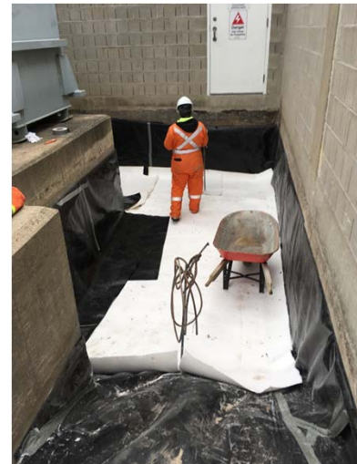
Installation of Oil Containment Solution
