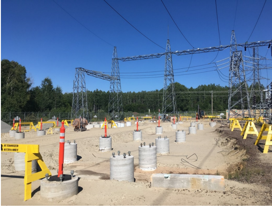
Wawa TS – Civil and foundation work underway
