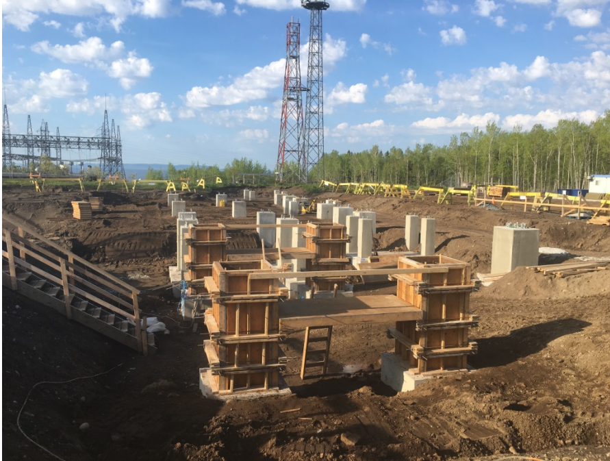
Lakehead TS – Civil and foundation work underway
