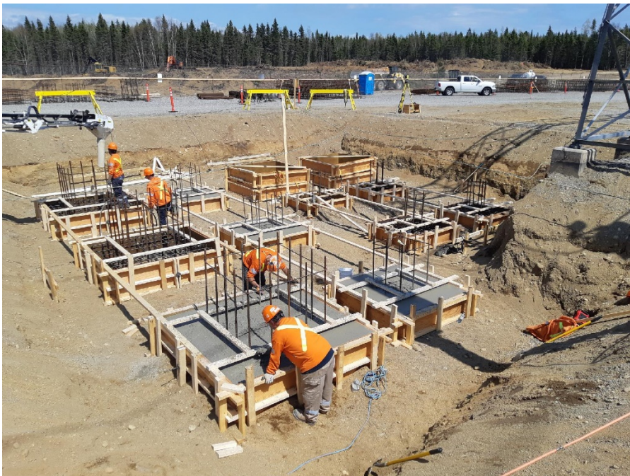
Marathon TS – Civil and foundation work underway
