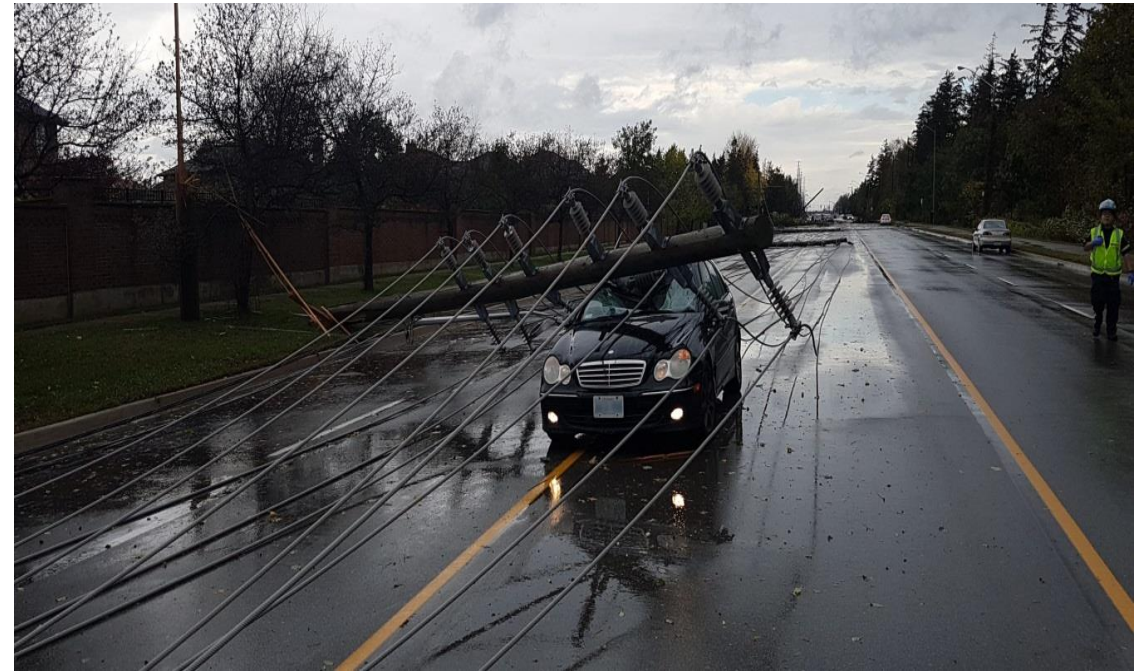
Failure of wood pole on October 15, 2017
