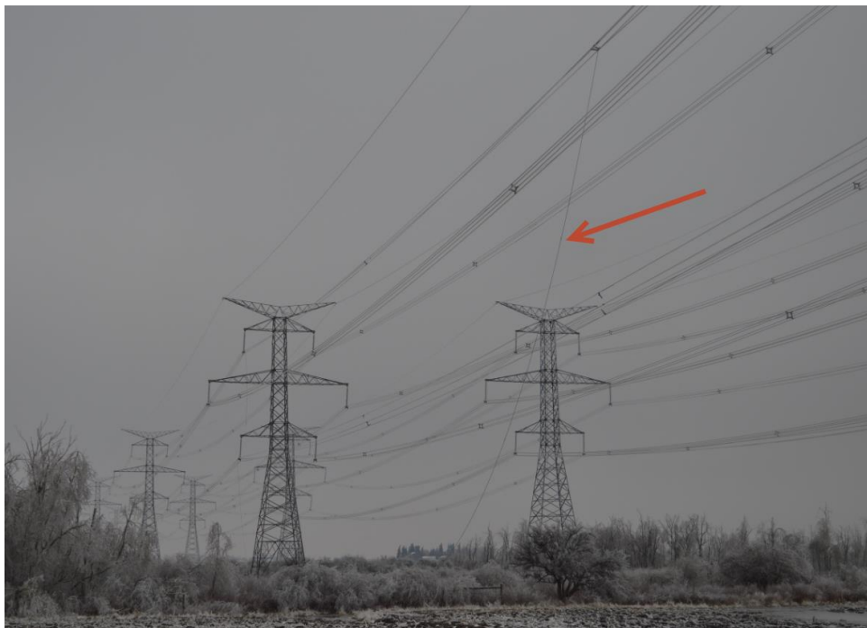
Figure 4 - Fallen span of conductor
