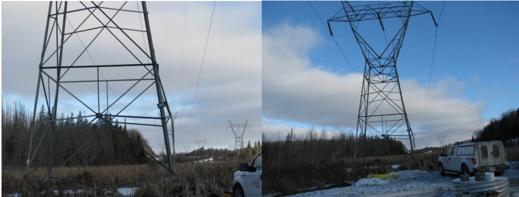
Figure 2 - Buckled legs and tower leaning (circuit M80B, Minden, ON)
