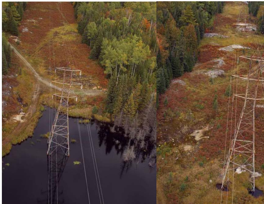
14 15 Figure 1 - Towers sitting in water causes the foundations to corrode, leading to 16 towers leaning (circuit D2L, near North Bay, ON)
