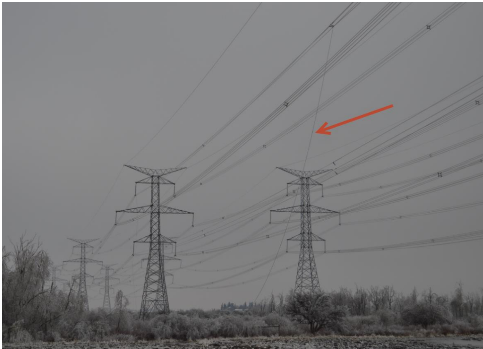
Figure 4 - Fallen span of conductor
