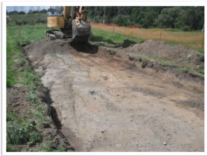
Figure 5: Photo depicting Gradall removing all topsoil from pathway location during URS Stage 4 Assessment. Assessment confirmed no features were present through monitoring and shovel shinning subsoil (URS Corporation, Stage 4 Mitigation (Avoidance and Protection) of the Parsons Site (AkGv-8) , April 2015).
