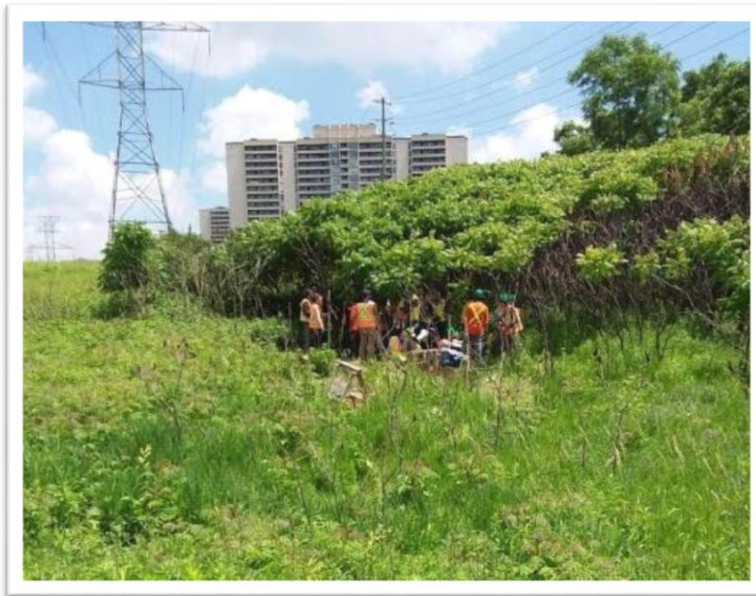
Figure 4: View of BH136 during Stage 2 testing, looking east. (The apartment building on Fountainhead Road is visible in the background. The watermain trench would be situated along the left hand edge of this photograph as the southern edge of the watermain trench is immediately north of the hydro tower.) (Past Recovery 2019)
