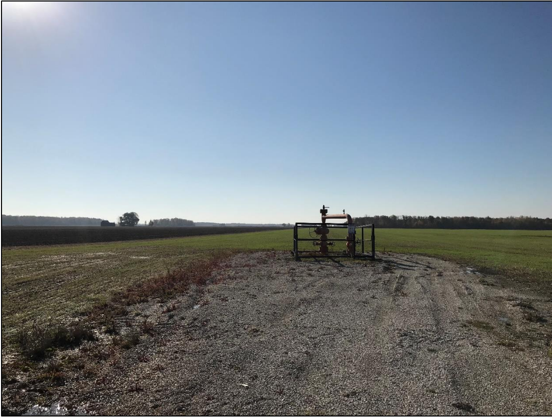
1. Temporary gravel pads are reduced following construction.
