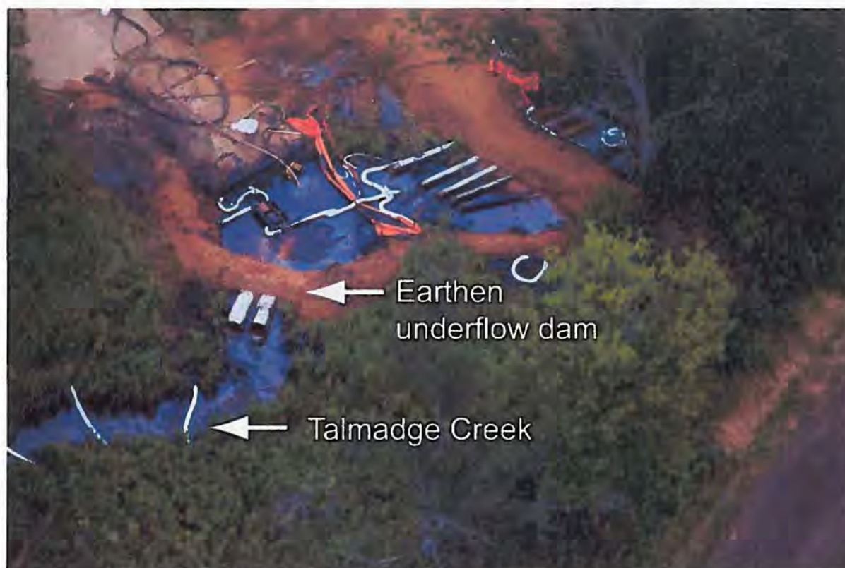
Figure 10. Underflow dam on Talmadge Creek on July 30, 2010.
