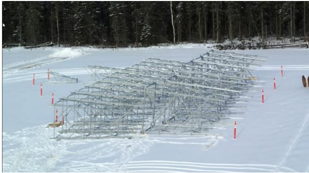
Marathon - Assembled Lattice steel sections
