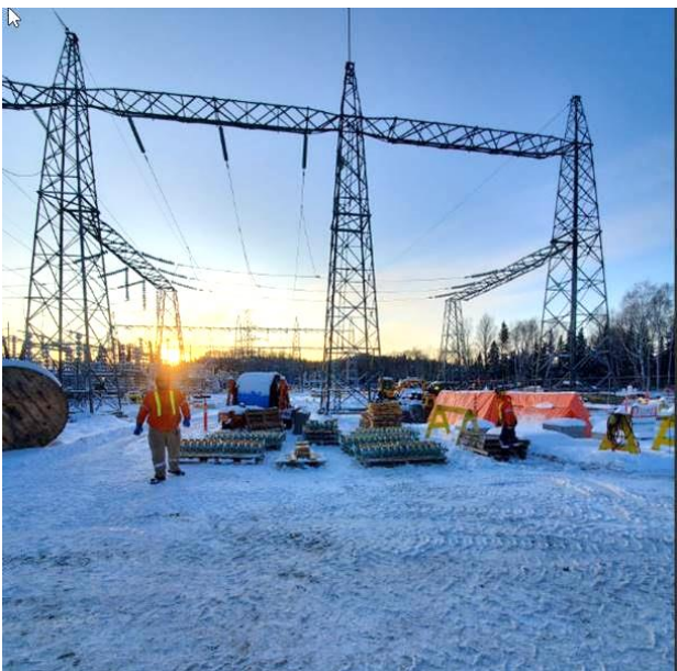
Wawa - Crews preparing for Bay 3 and Bay 4 new strain bus installation:
