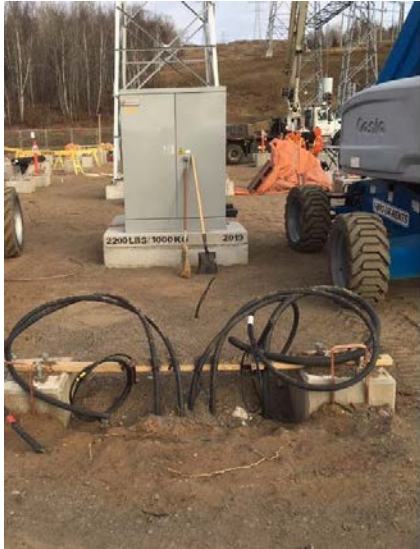
AC TF-SS installed and cables pulled to new AC panel board and safety switch location
