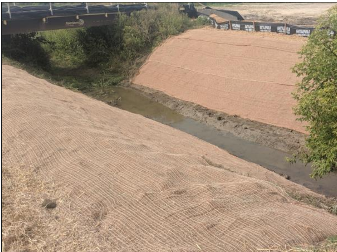
6. Sediment and erosion control measures were installed at each watercourse crossing and will remain in place until the banks are stable and vegetated.
