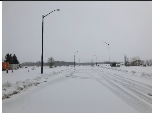
Innisvillage Subdivision Construction
