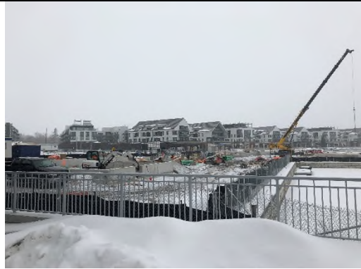
Friday Harbour Resort Construction
