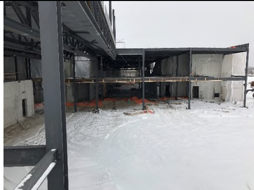
Secondary School Construction
