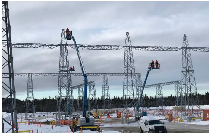
Marathon - Bay 6 & 7 securing lattice steel
