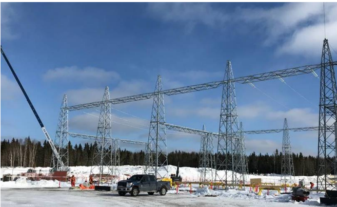
Marathon - Bay 5 & 8 strain bus span install
