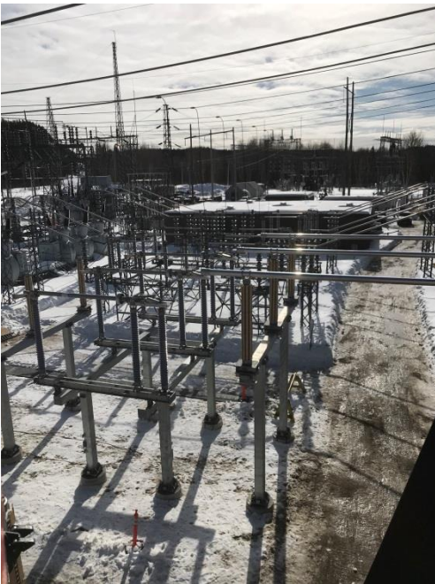
Wawa – Bay 3 & 4 bus & switch support structures
