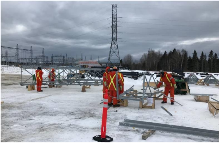
Marathon – Assembling lattice steel for Bay 7
