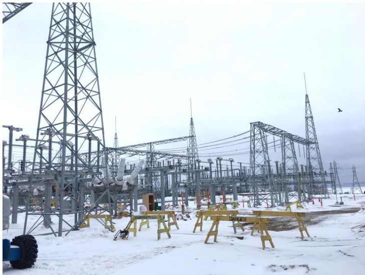
Lakehead - Side view of Bay 9 and 10 with new cable trench
