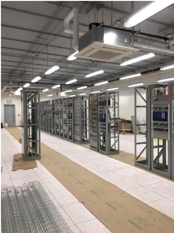
New 230kV building rack installation
