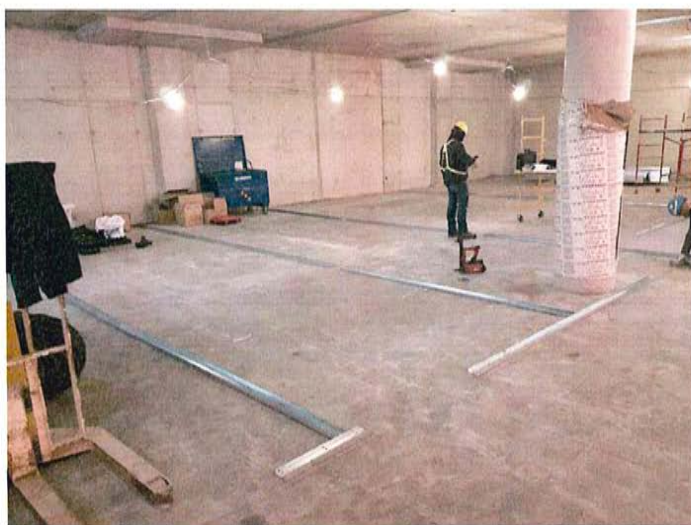
EC1 Interior Wall Framing LO (January 018)
