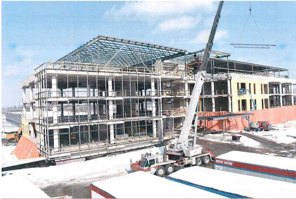
EC1 Exterior Wall and Window Framing & Sheathing (January 018)
