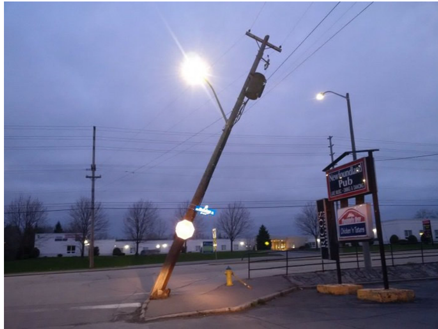
Figure 3: The X23085 broken pole on 940 Montreal Road
