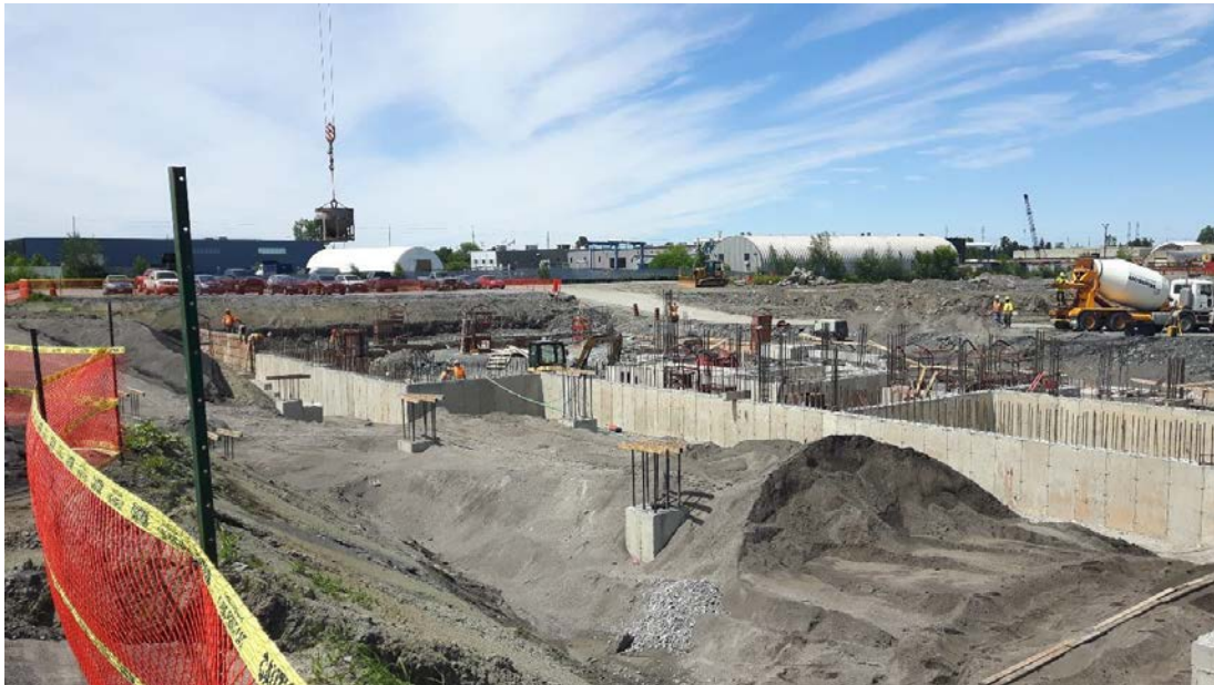
EC1 foundation wall concrete placement and backfilling
