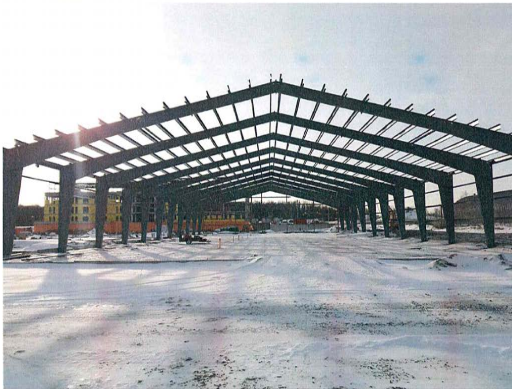
EC2 Pre-engineered Garage Steel erected
