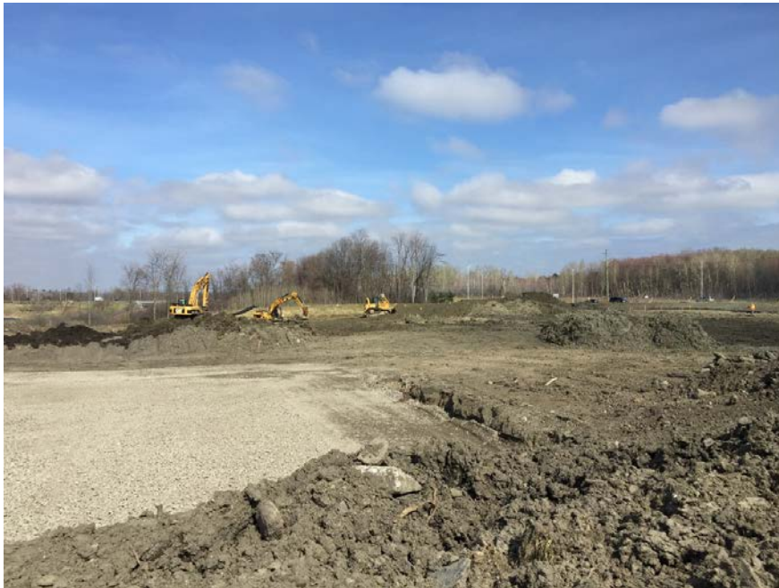
East Campus – Excavation and placement of granular pad for EC2
