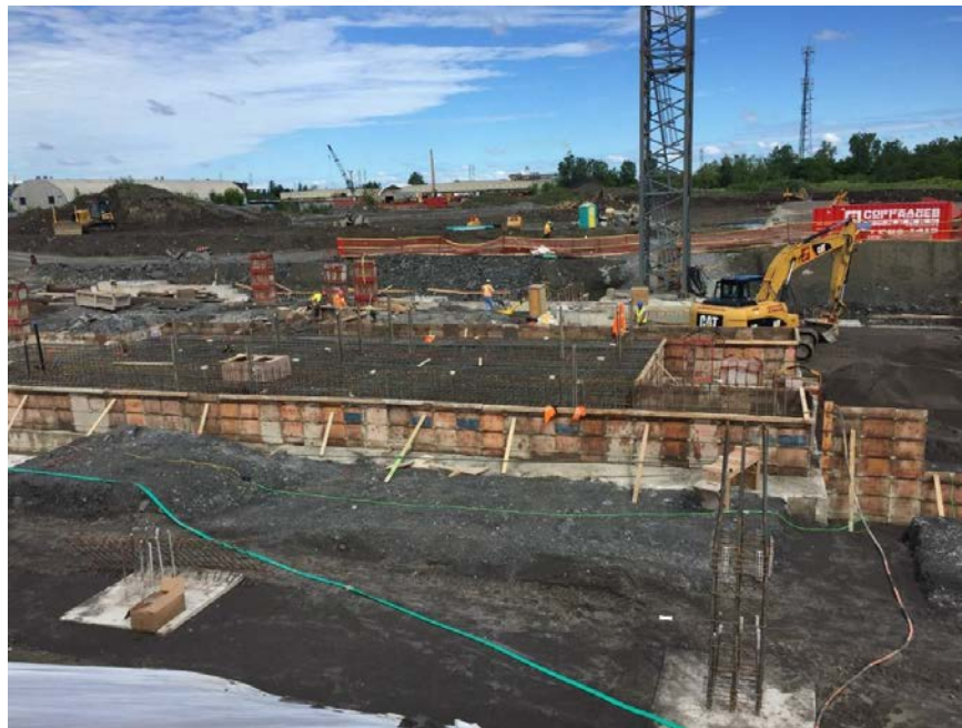
EC1 raft footing at East end of building
