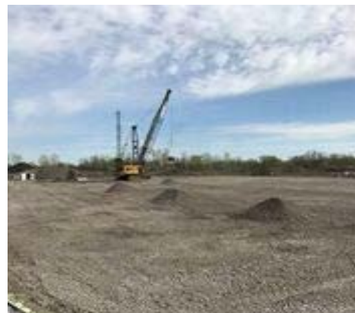
EC2 Dynamic compaction
