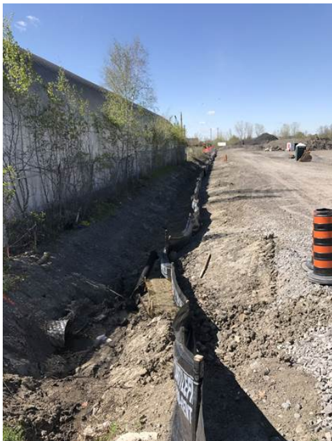
STW drainage swale - west
