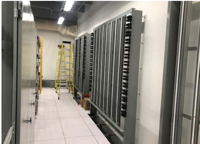
Marathon – 'A' room terminal racks installed in PCT building
