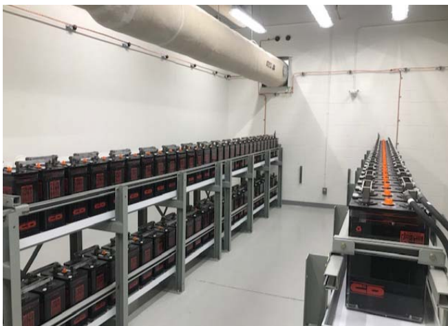
Marathon – 'B' battery racks in PCT
