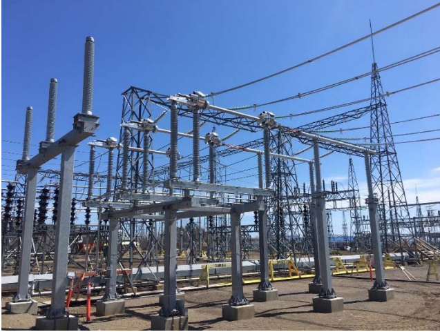
Lakehead - Bay 9 & 10 new lattice steel structures and towers
