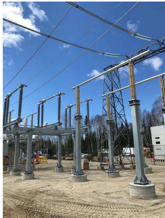
Wawa – Bay 3 & 4 bus & switch support structures
