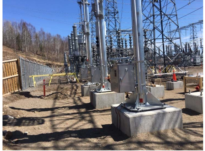
Lakehead - Bay 9 and 10 new bus support structures/switch structure
