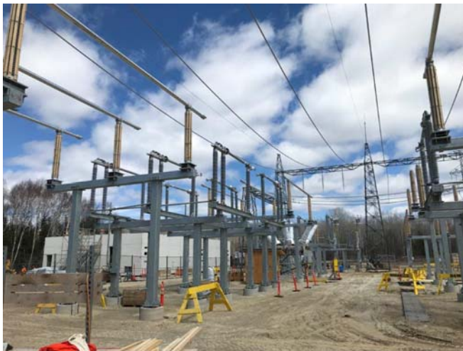
Wawa – Bay 3 & 4 bus & switch support structures
