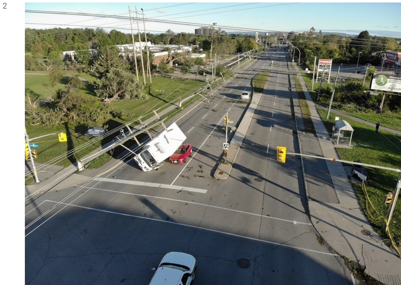
1 Figure 4.21 – Downed Pole Line Following September 2018 Tornado Event
