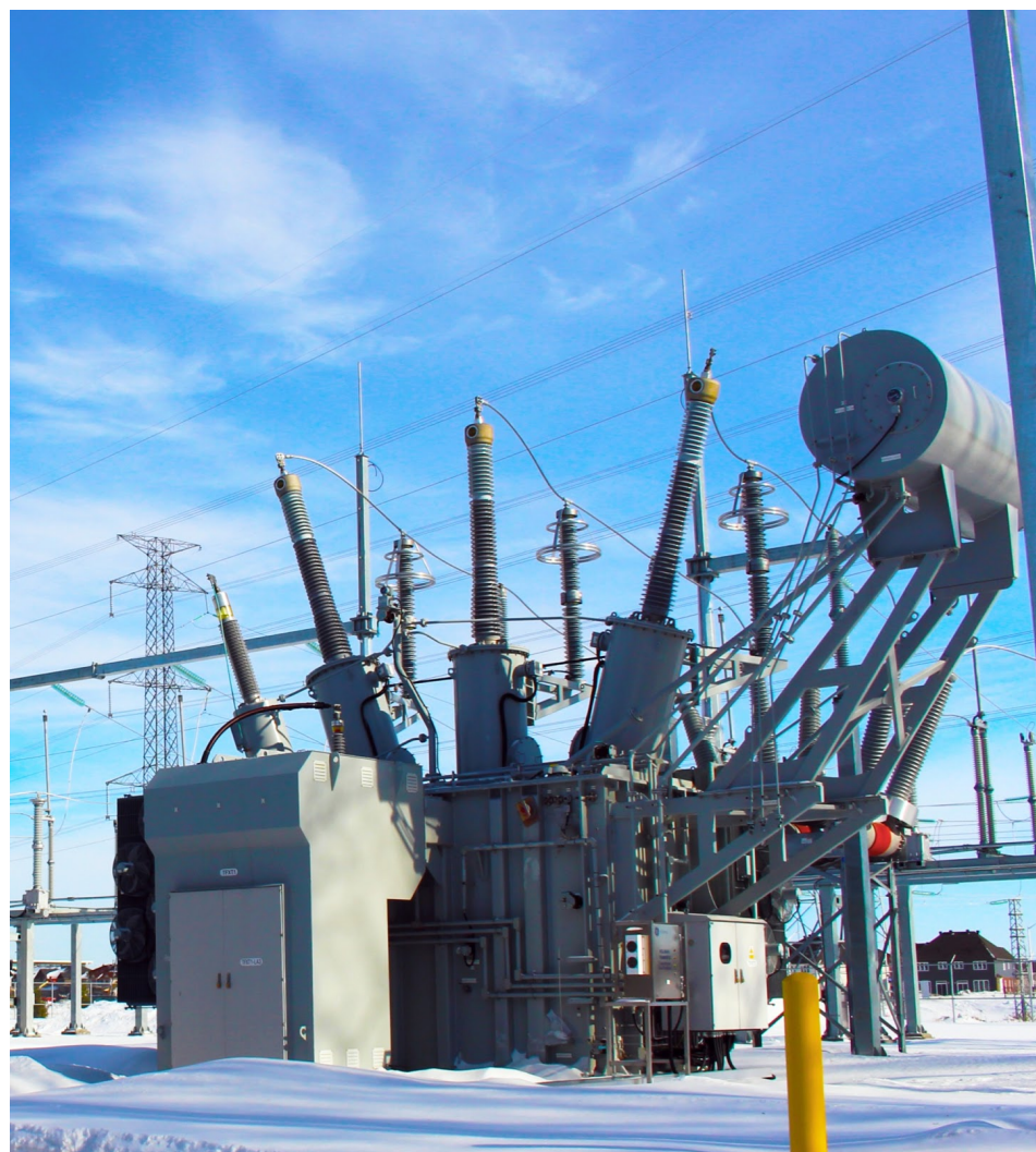
Figure 4.9 – Station Transformer at Terry Fox MTS
