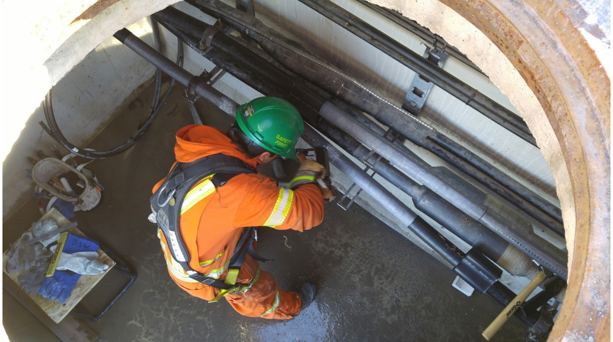
Figure 6.48 – Cable Splicing within a Cable Chamber
