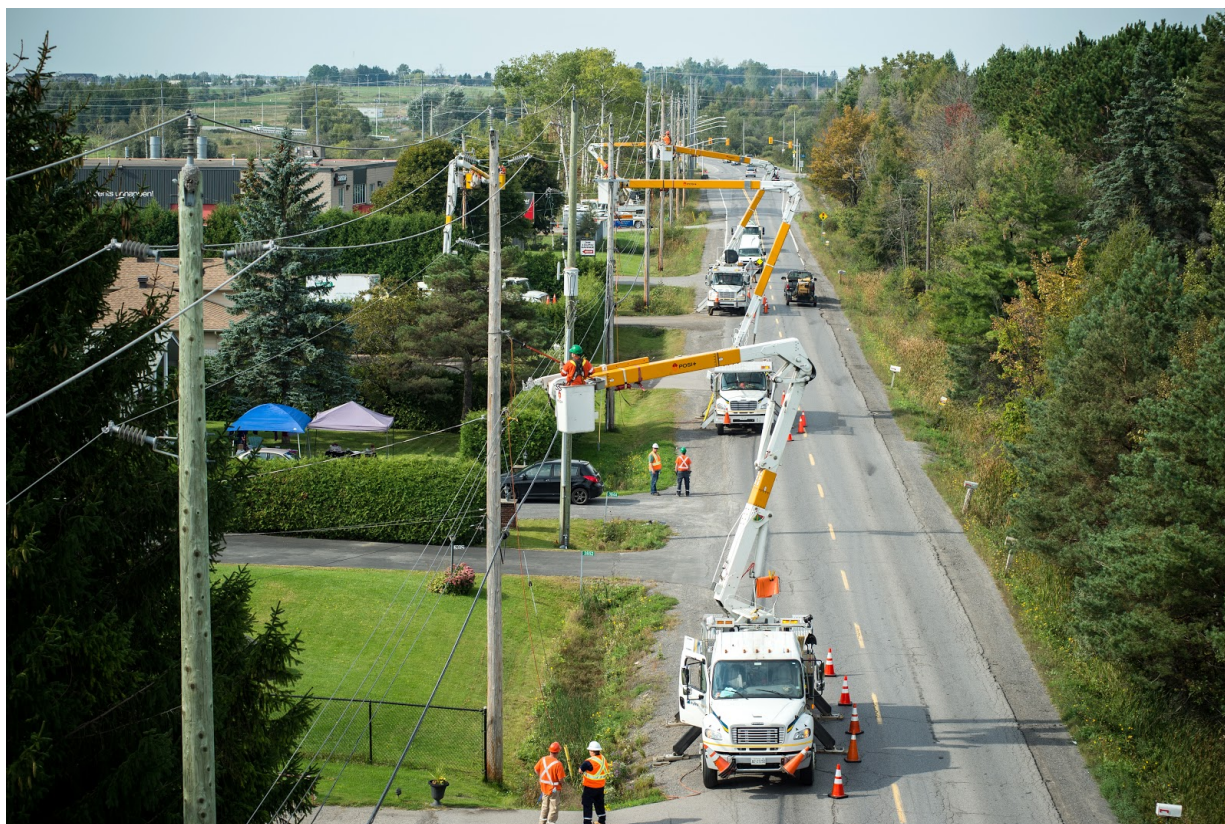
Figure 1.2 – Planned Insulator Replacement on 27.6 kV Pole Line
