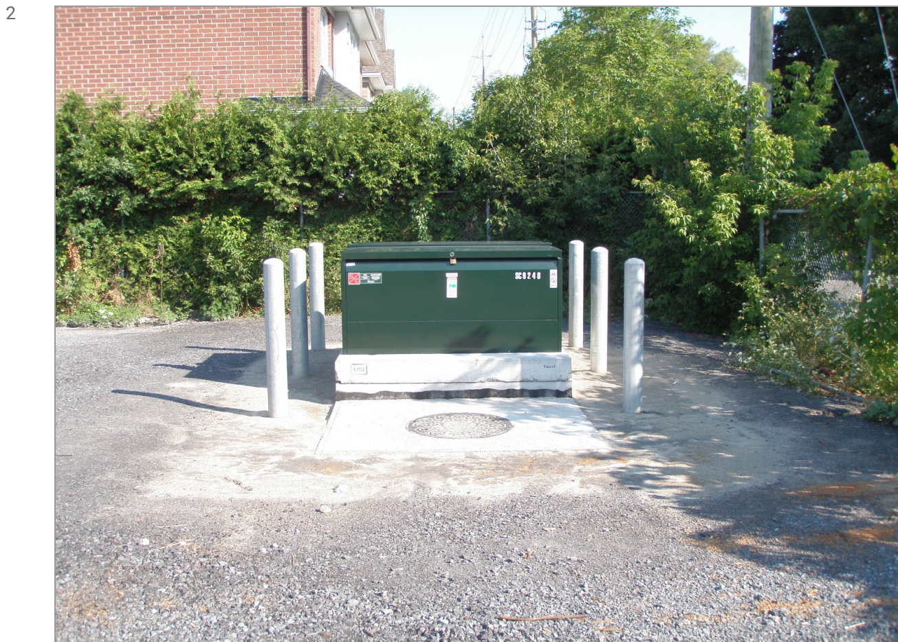
1 Figure 6.42 – Typical Installation of a Vista Type Underground Switchgear
