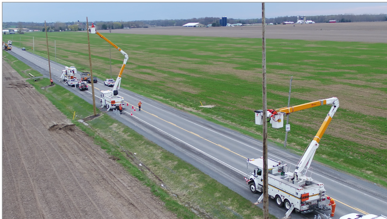
Figure 6.22 – Installation of New Pole Line
