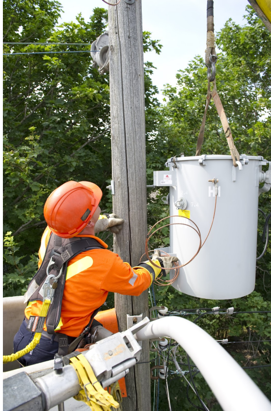
Figure 6.26 – Installation of Overhead Transformer
