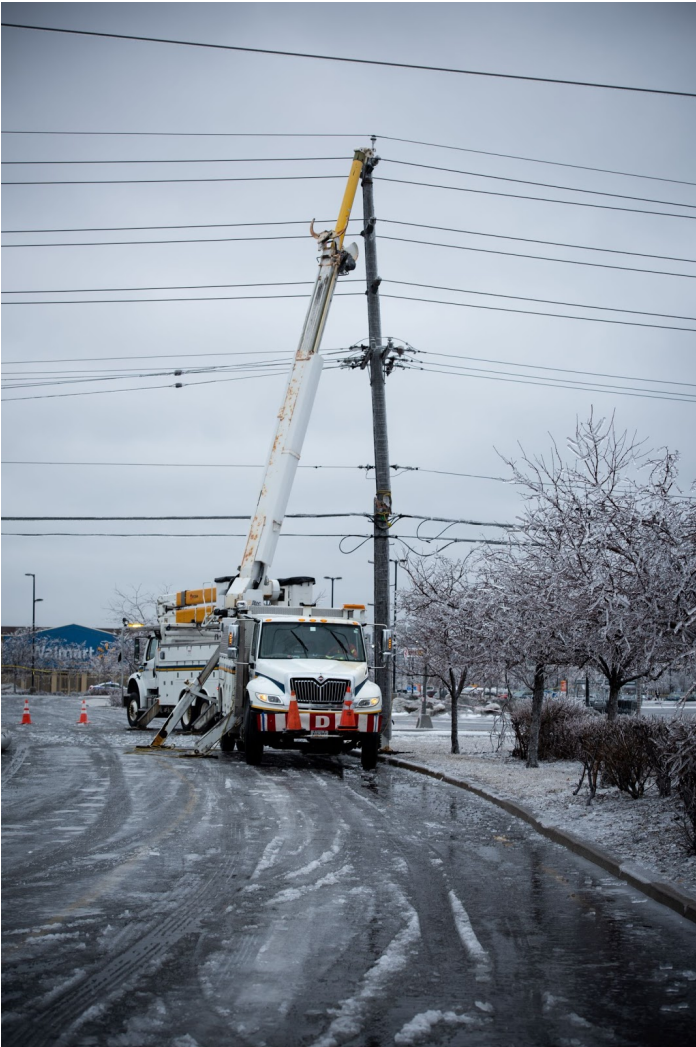
Figure 2.9 – Pole Replacement Following 2018 Ice Storm
