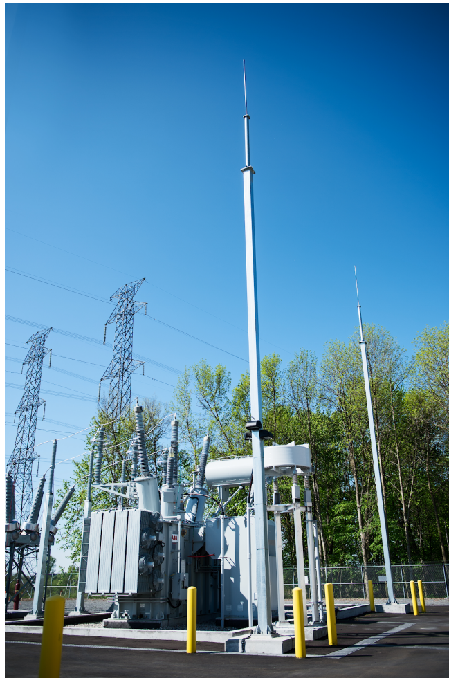
Figure 6.5 – 28 kV Station Transformer at Terry Fox MTS
