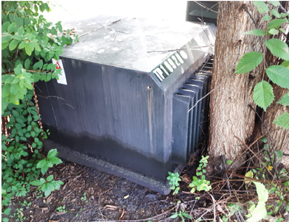
Figure 4 – Leaking Transformer
