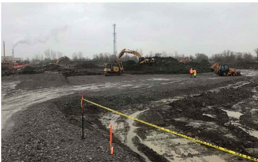
East Campus – Excavation and placement of granular pad for EC2
