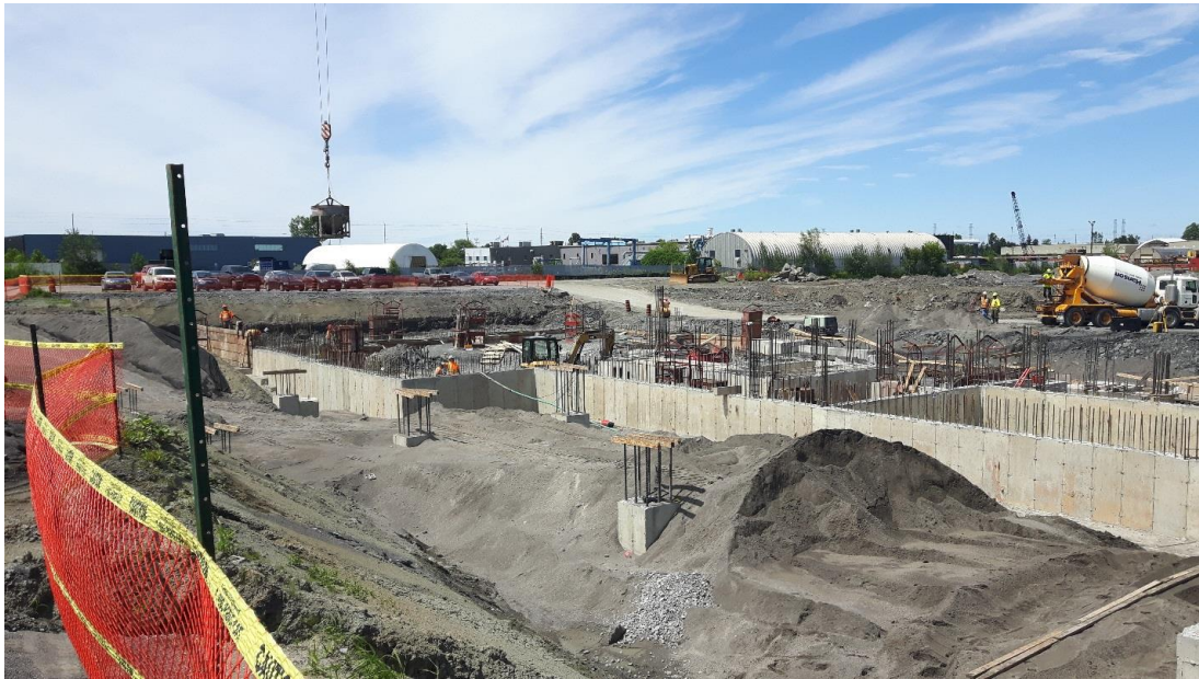
EC1 foundation wall concrete placement and backfilling
