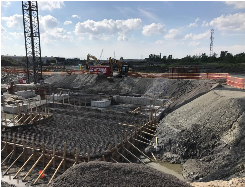
EC1 raft footing at East end of building
