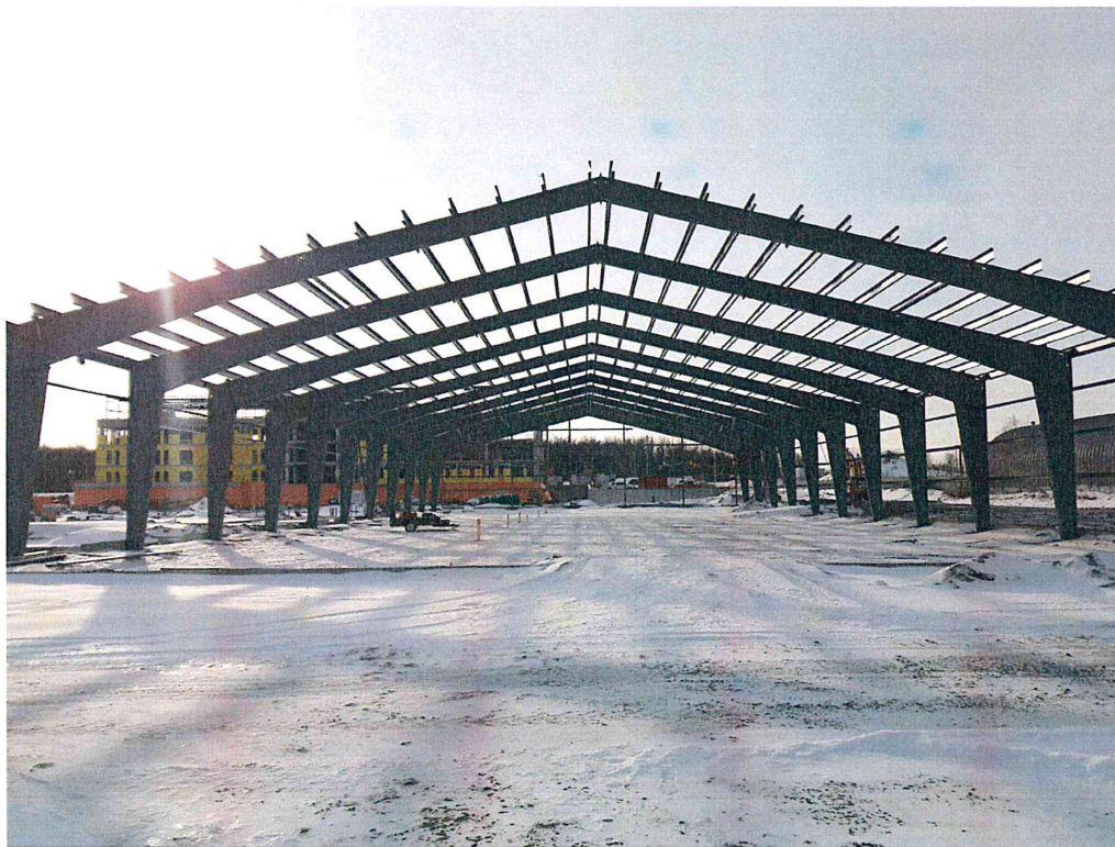
EC2 Pre-engineered Garage Steel erected
