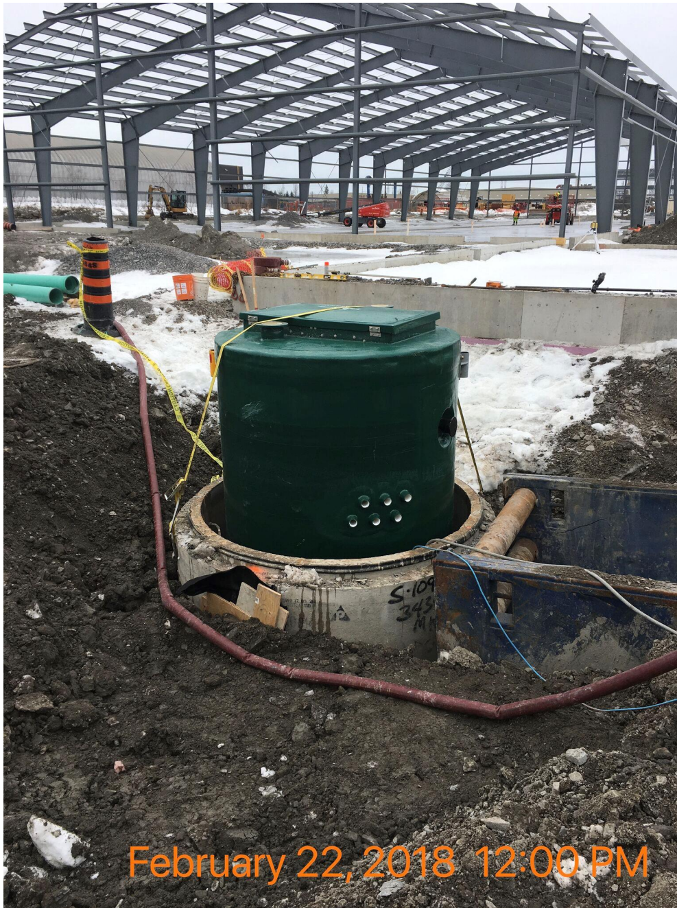
EC Sanitary pumping station
