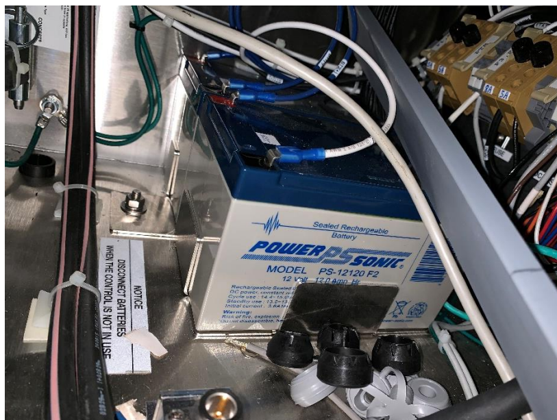
Figure 72- Example of a battery used
