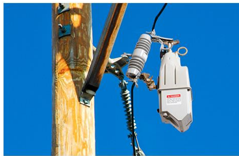
Figure 49- Lateral recloser
