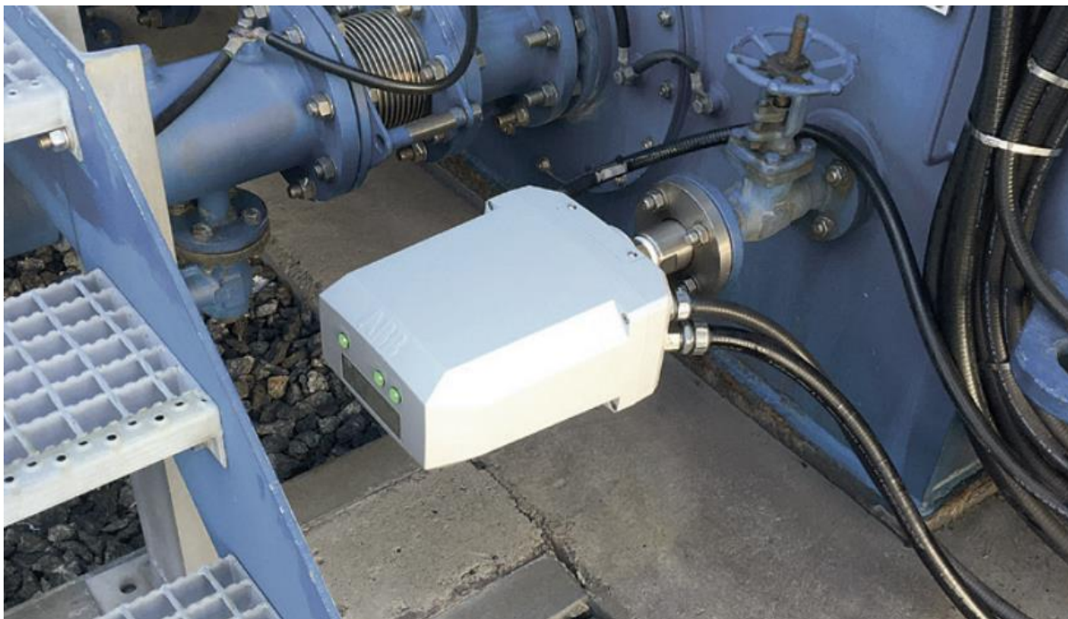
Figure 35 - Example 2 of Transformer Monitoring Device Installed
