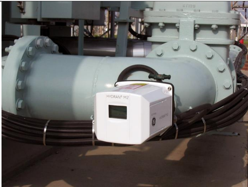
Figure 34- Example of Transformer Monitoring Device Installed
