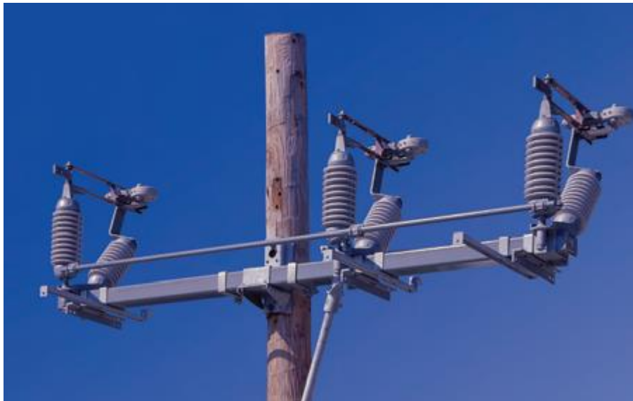
Figure 43- Remote 44kV Switch
