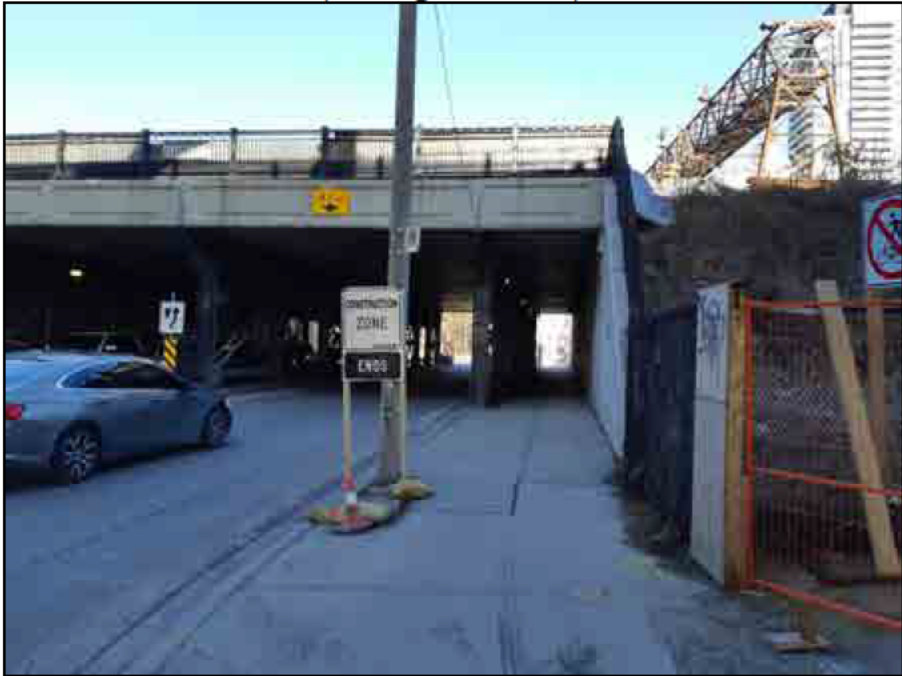
Image 7: Parliament Street at Lake Shore Boulevard (looking northwest)
