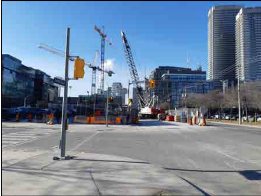
Image 12: Queens Quay at Lower Sherbourne Street, Southern ROW (looking southwest)
