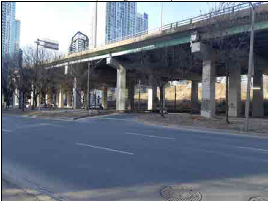
Image 42: Lake Shore Boulevard east of Dan Leckie Way (looking northwest)
