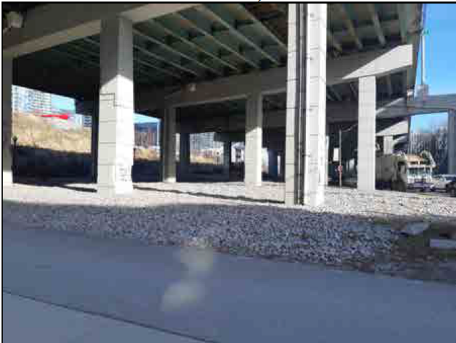
Image 40: Lake Shore Boulevard at Dan Leckie Way (looking northeast)
