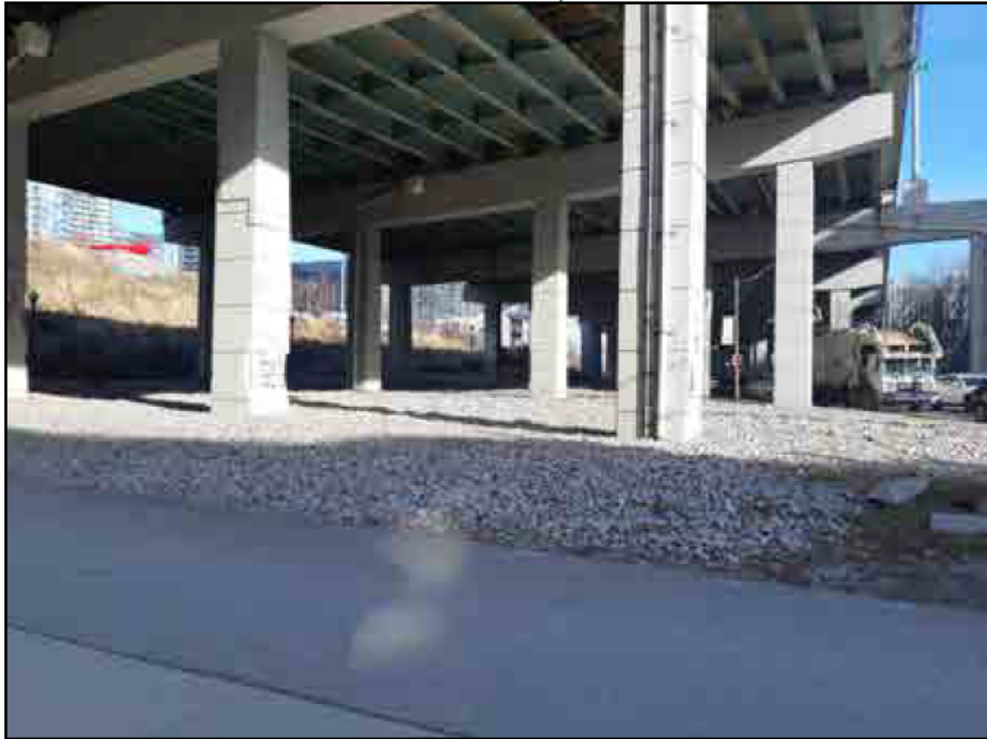
Image 35: Lake Shore Boulevard at Spadina Avenue (looking northeast)
