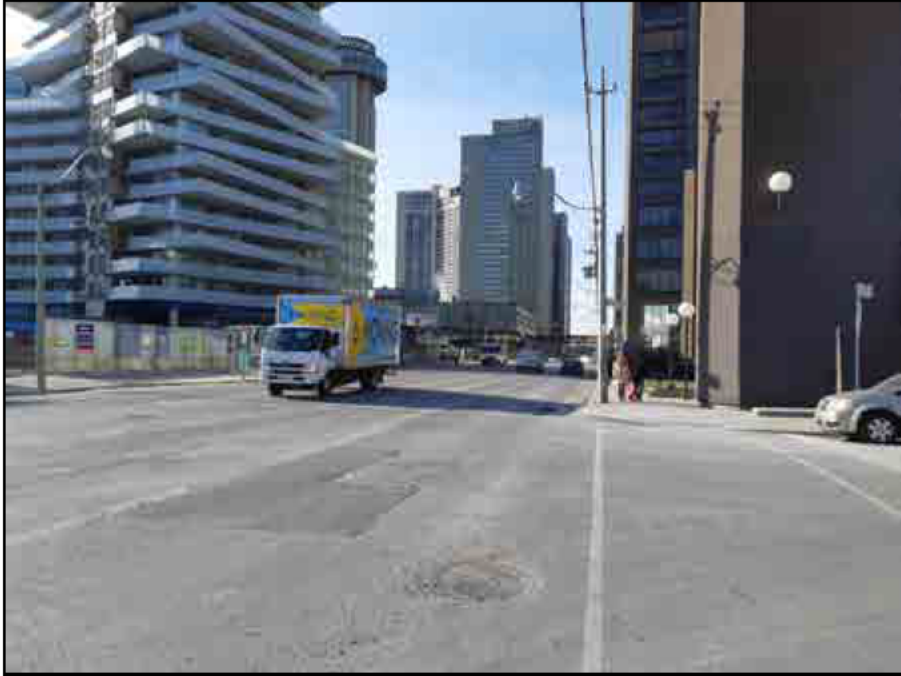
Image 22: Queens Quay at Freeland Street, Northern ROW (looking southwest)
