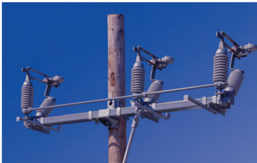
Figure 43- Remote 44kV Switch
