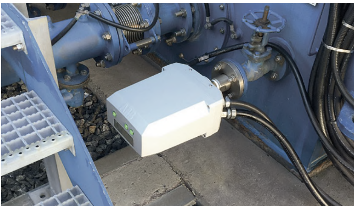
Figure 35 - Example 2 of Transformer Monitoring Device Installed
