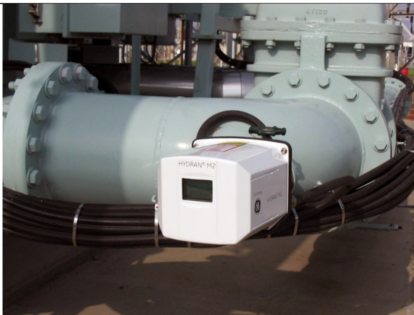
Figure 34- Example of Transformer Monitoring Device Installed
