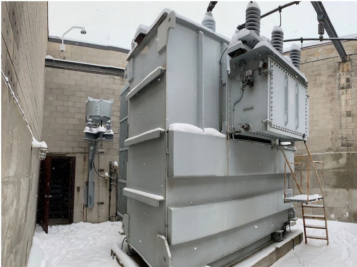
Figure 32- Photo of a Municipal Substation Transformer
