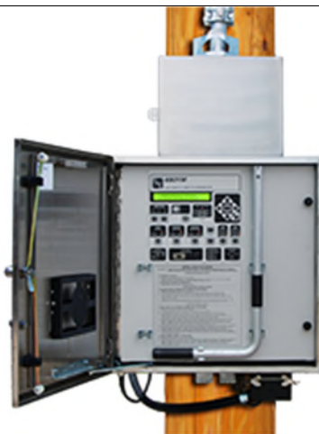
Figure 44-Motorized Controller of 44kV Switch
