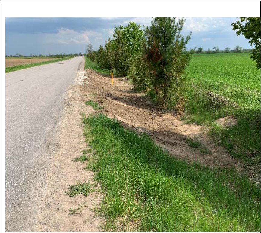
Photo 5: Road ditch between Flos Road 6 and Flos Road 5.
