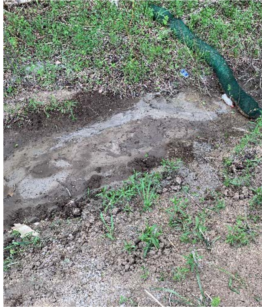
Photo 4: Silt Soxx™ limiting potential for off-site sedimentation between Flos Road 7 and Flos Road 8.
