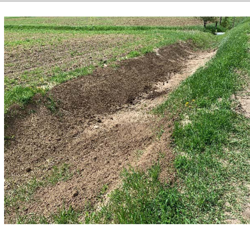
Photo 6: Reclaimed ditch between Flos Road 5 and Flos Road 4.
