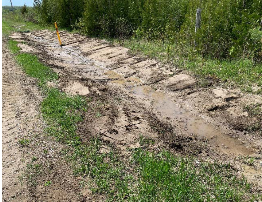
Photo 1: Soft ditch on Flos Road 8, reclaimed and seeded.
