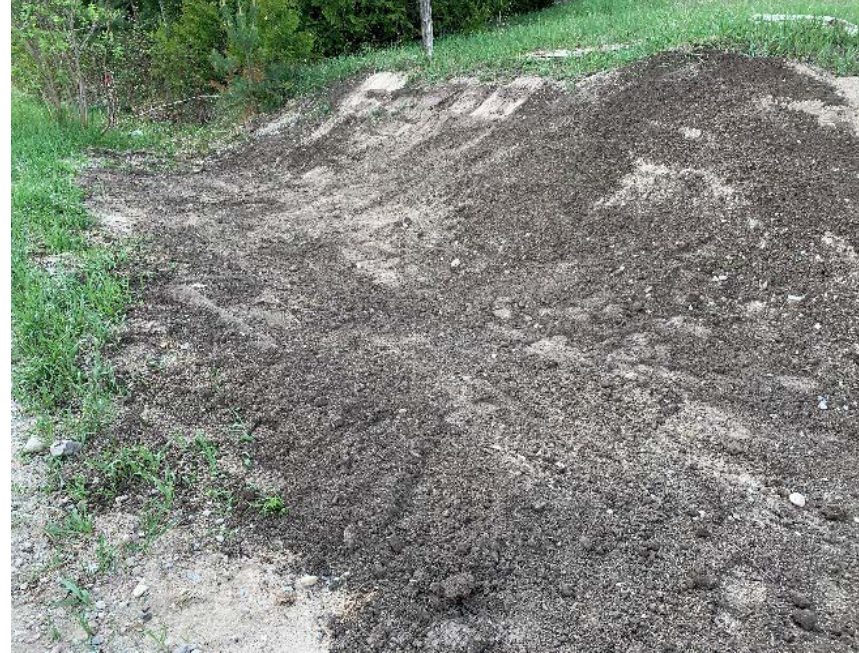
Photo 2: Sandy embankment on Flos Road 8 which has topsoil and seed applied.
