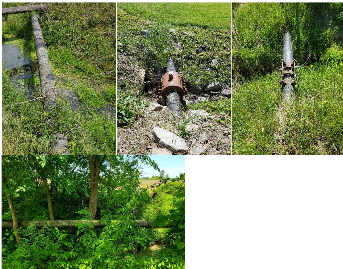
Figure 4-1 Examples of London Lines Exposed Piping (June 2020)
