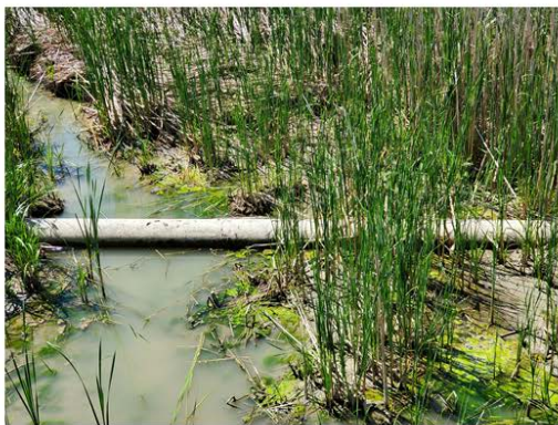
Figure 5: Aerial Crossing near municipal drain, potential for pipe to be partially submerged (Mossie Line, West of Burr Rd). Left is a close-up, right show the crossing in context.
