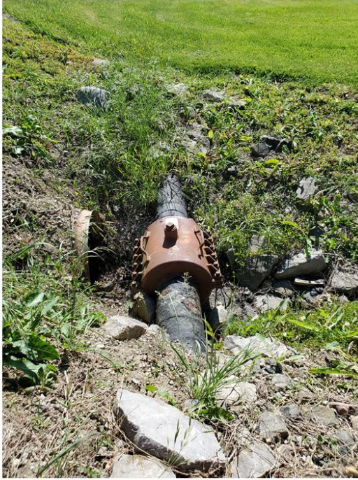
Figure 1: Aerial Crossing with Mechanical Split Sleeve Repair fitting, covering leaking Dresser Coupling, near municipal culvert, Bentpath Line, west of Marthaville Rd). Left is a close-up, right show the crossing in context.
