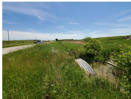
Figure 5: Aerial Crossing near municipal drain, potential for pipe to be partially submerged (Mossie Line, West of Burr Rd). Left is a close-up, right show the crossing in context.
