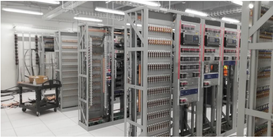
Marathon – ‘B’ room terminal racks installed in PCT building
