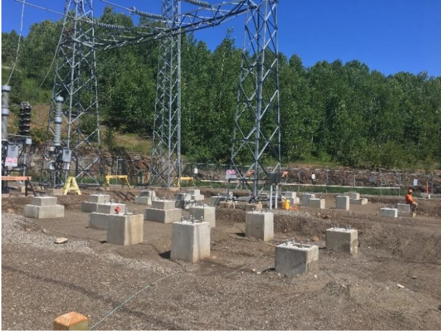
Lakehead – new footings for yard expansion
