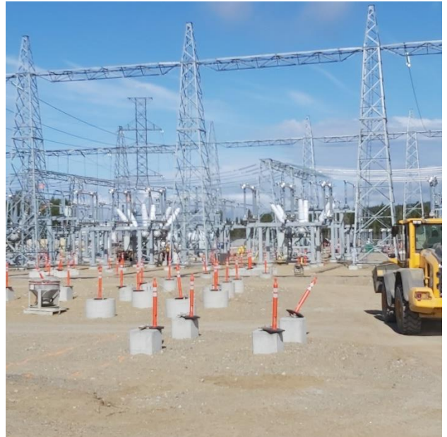
Marathon – Footings for phase 2
