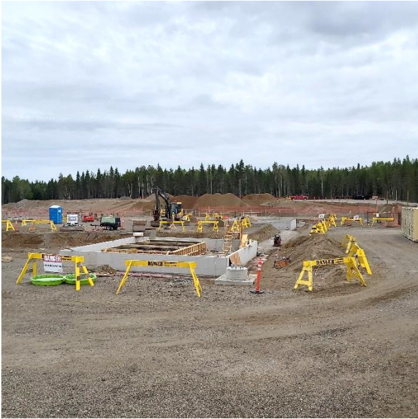
Marathon – Reactor spill pits for R3 & R4
