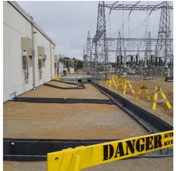
Marathon – Cable pulling from PCT building to external equipment
