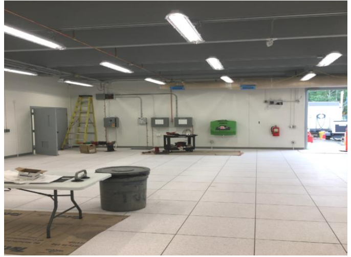
Wawa – Inside PCT building
