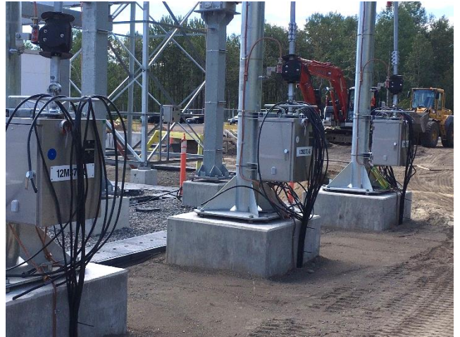
Lakehead – Various mechanical boxes being wired
