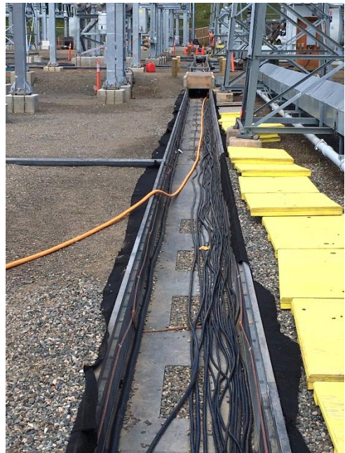
Lakehead – Field cable pulling throughout
