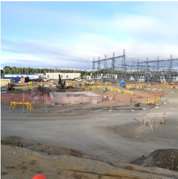
Marathon – Yard expansion overview
