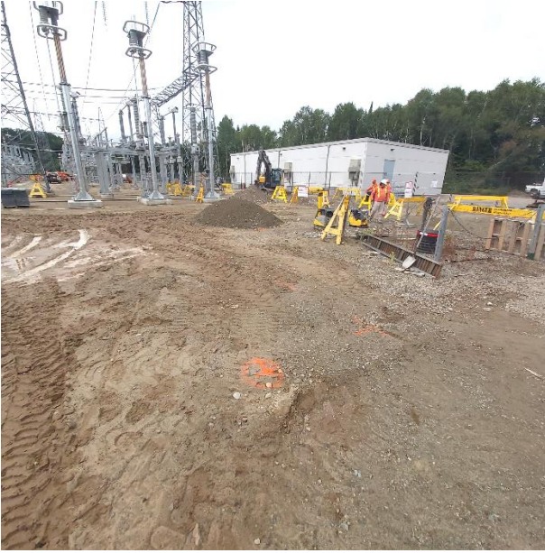
Wawa – Bay 4 tower & PCT building
