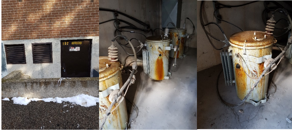
Figure B.1-9: The transformer vault door and transformers within.
