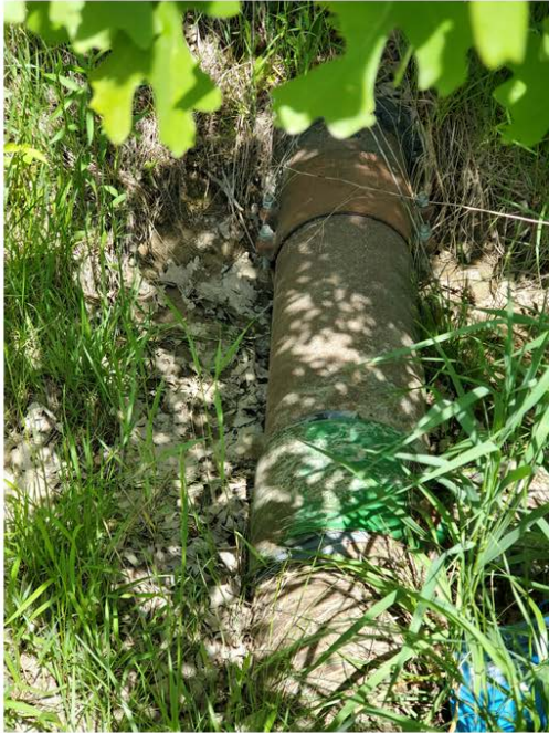
Figure 7: Aerial Crossing with multiple leak repair clamps over corrosion leak on pipe (Old Airport Rd, north of CPR Dr). Left is a close-up, right show the crossing in context.
