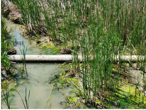
Figure 5: Aerial Crossing near municipal drain, potential for pipe to be partially submerged (Mossie Line, West of Burr Rd). Left is a close-up, right show the crossing in context.
