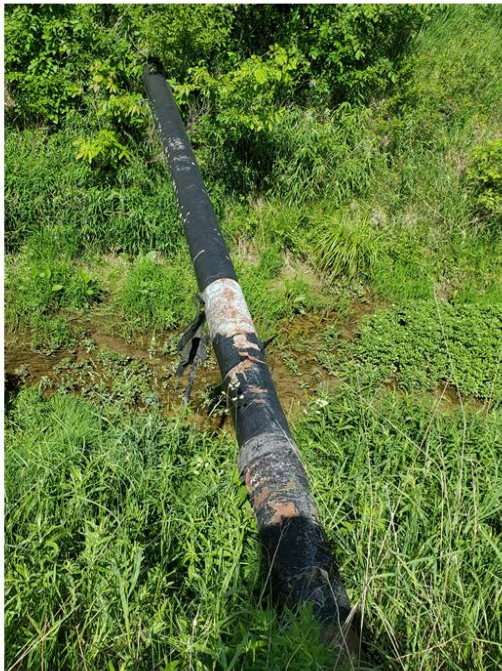
Figure 8: Aerial Crossing with pipe coating peeling off (Falconbridge, between Tait's Rd and McArthur Rd). Left is a close-up, right show the crossing in context.
