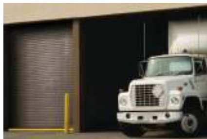
Figure 2 Example of "Drive-in" Shipping and Receiving doors 2
