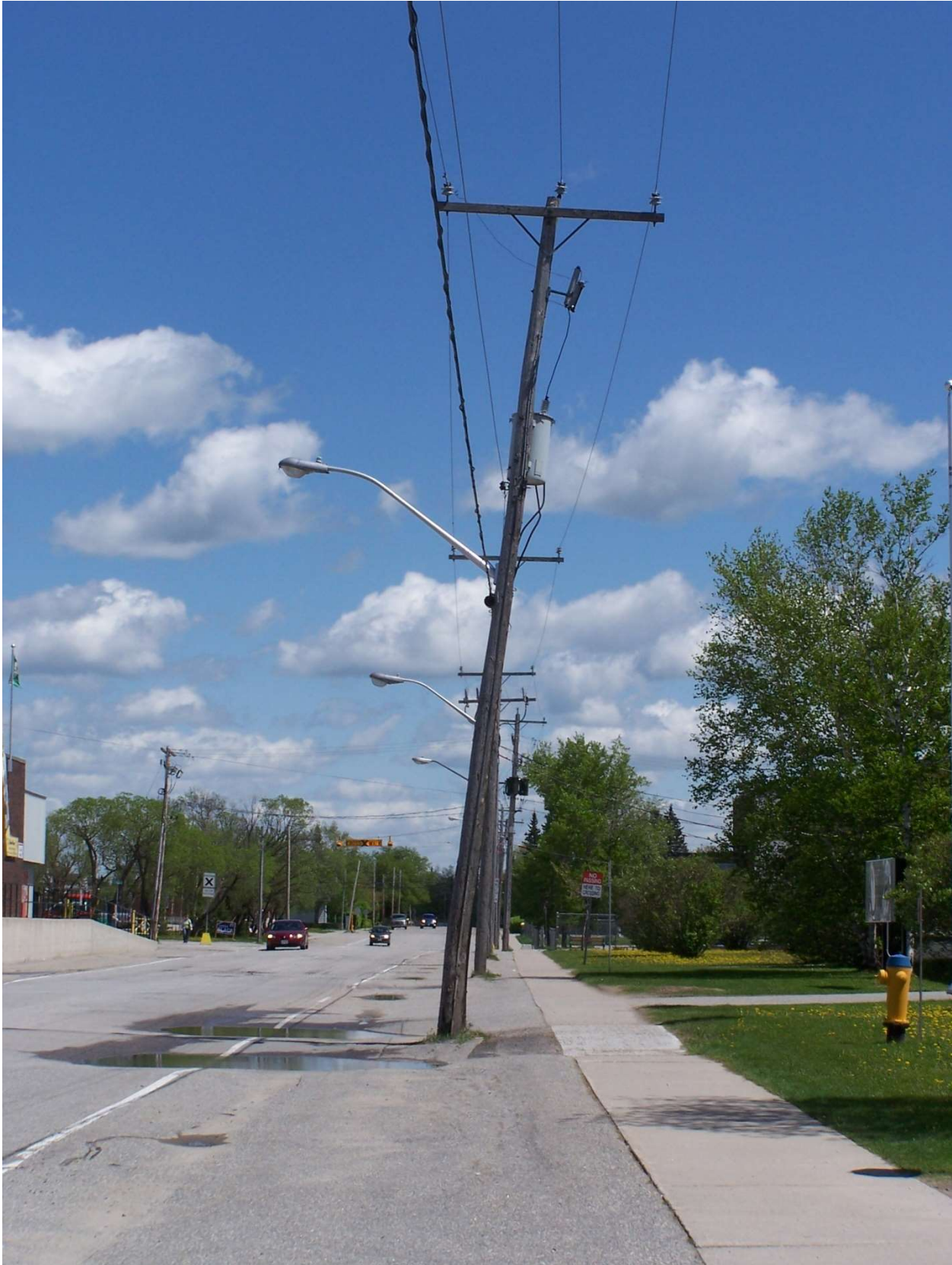
Pole deforming due to reduced fiber strength and side force loading
