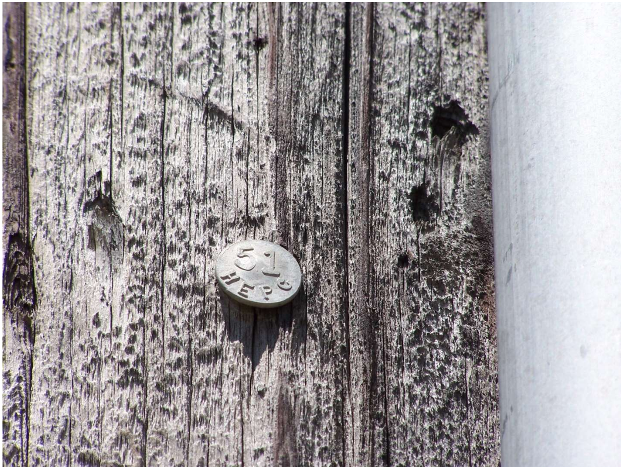
An "old" pole- installed in 1951
