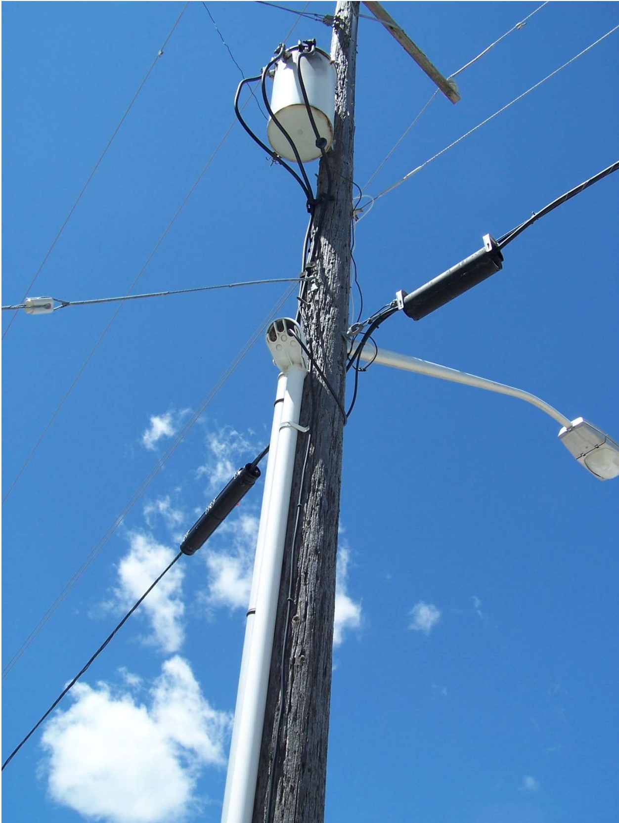
An example of wood fiber deterioration
