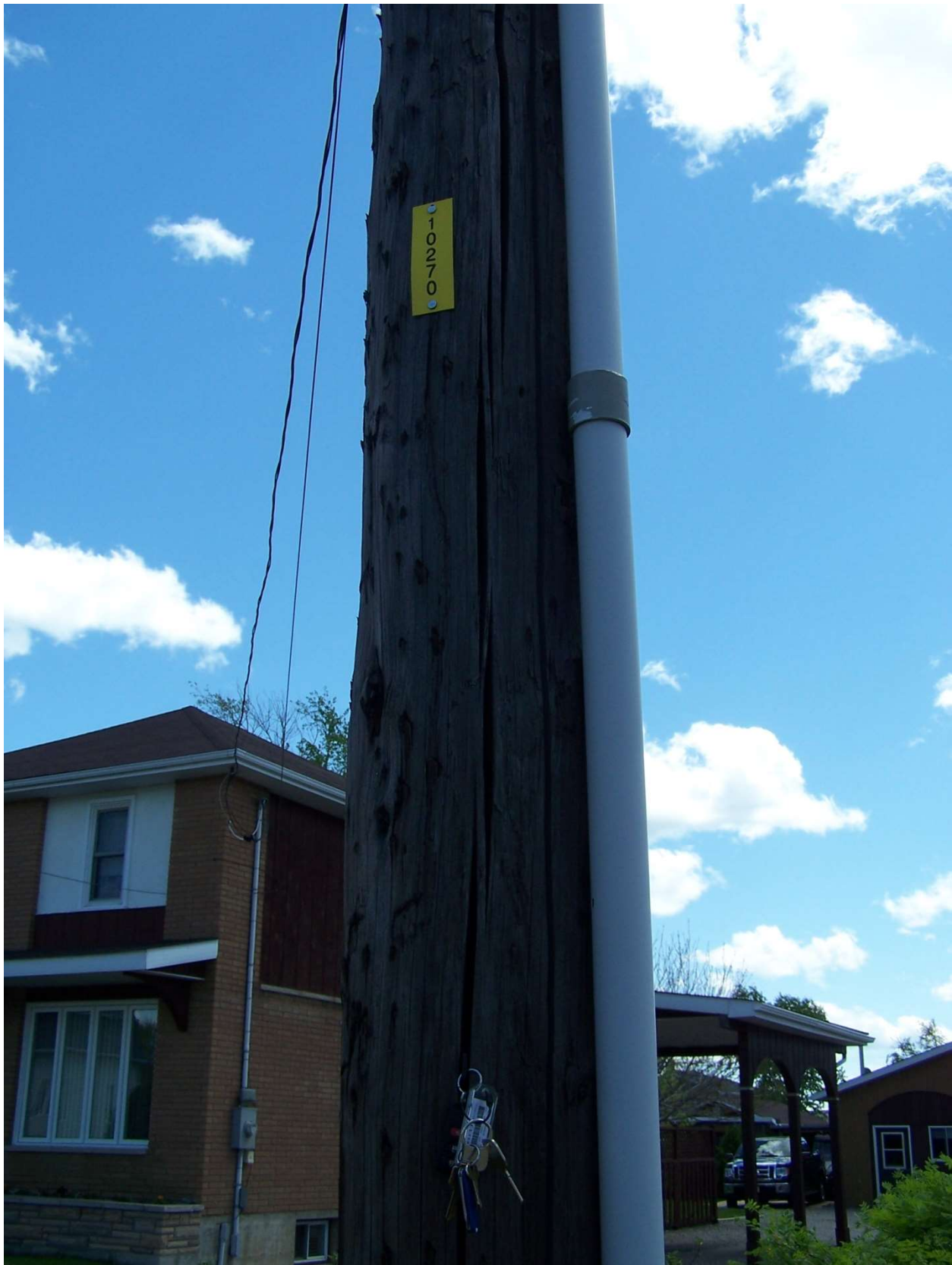
An example of long deep cracks
