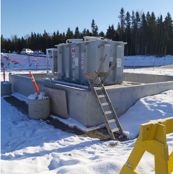
Marathon – Reactors R3 & R4 install
