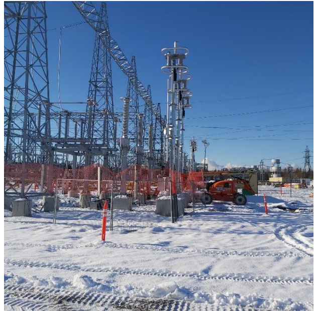
Marathon – CVT's and arrester install
