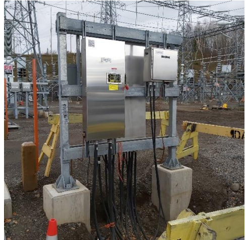
Lakehead – AC station service and Auto Transfer scheme
