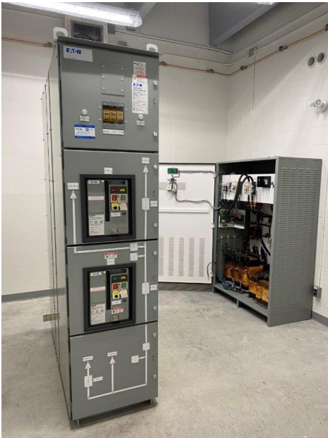
Wawa – 'A' charger and switchgear
