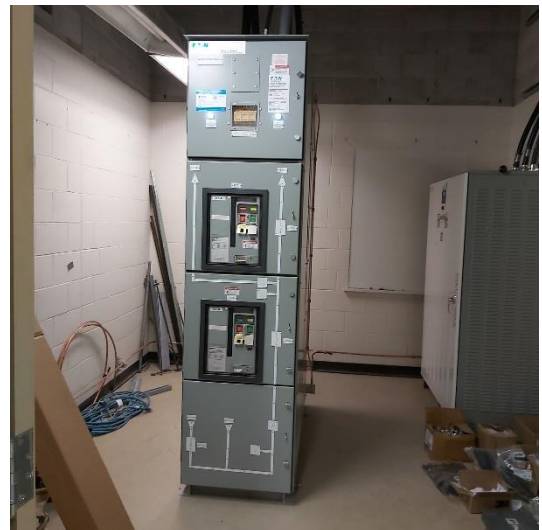
Lakehead – DC switchgear in existing Control Building
