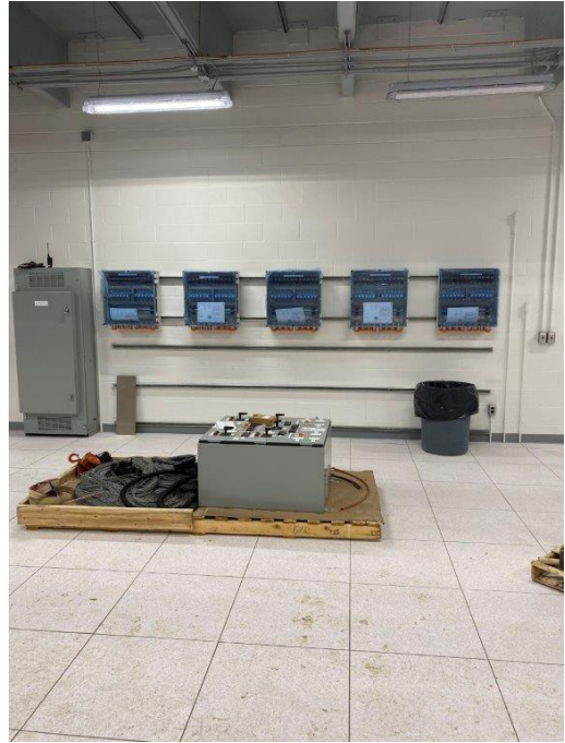
Wawa – "B" DC monitoring cabinets installed
