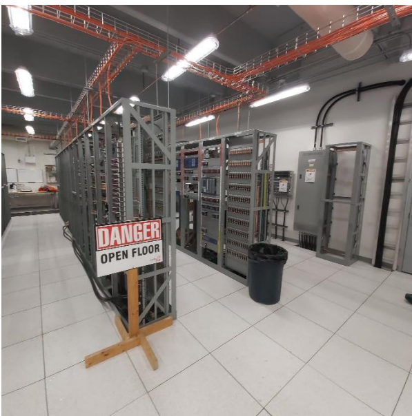
Marathon – Various fiber tray above racks for communications
