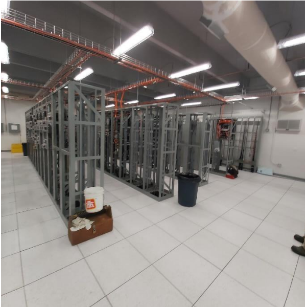
Marathon –Completed all internal cable pulling and terminating
