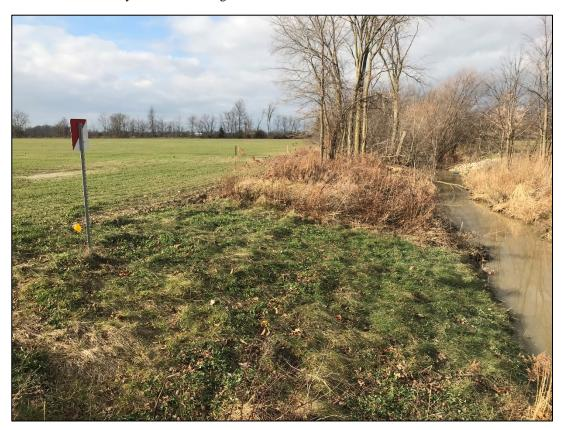
2. Watercourse crossings are monitored the year following construction and if the banks are stable and re-vegetated, erosion control measures can be removed.
