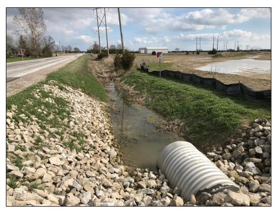
3. Rip-rap is used in select areas for additional stability on steep banks along roadsides. Clean-up work could also not continue until soils were dry.
