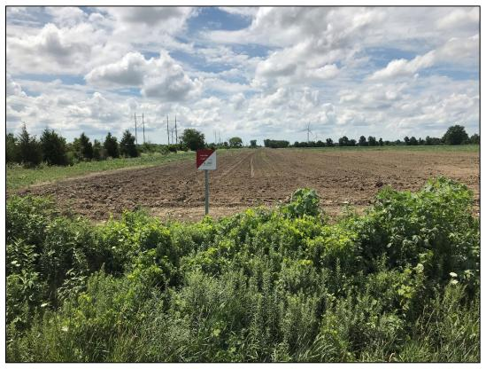
4. Once the topsoil is restored back to agricultural fields, stones and debris are picked and the soil is disked, decompacted, and re-graded.
