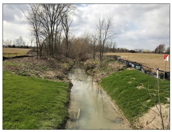
1. Silt fencing and erosion control measures are left in place around watercourse crossings until the banks are fully stable and re-vegetated.
